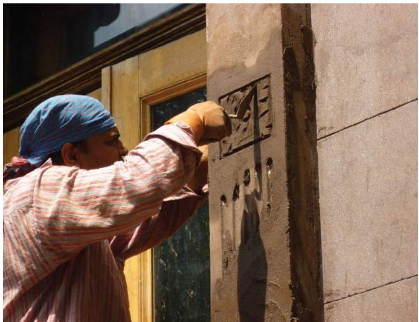
Resurfacing ornament with cementitious brownstone-tinted stucco to replicate historic details.
