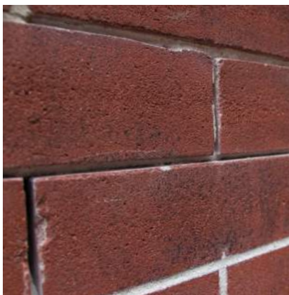
An example of careful mortar joint removal.
