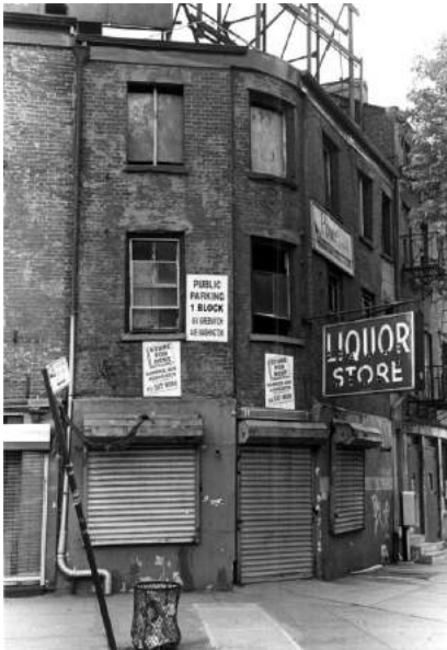
Before facade reconstruction.
