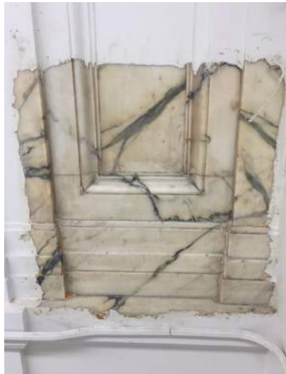
Coating removal without damaging the historic material
