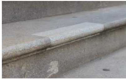
The light colored stone seen on the lower step is replacement stone installed as a Dutchman repair.
