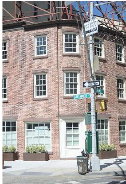
After facade reconstruction.
