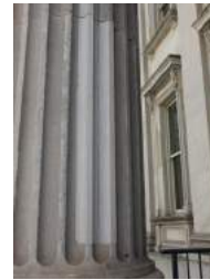
The light colored stone shown here is replacement stone installed as a Dutchman repair.
