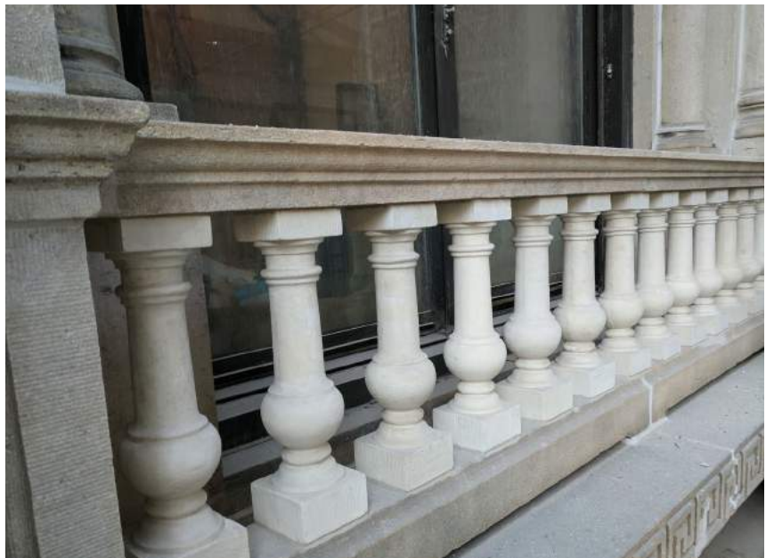
Replacement balusters that match the historic ones in terms of their dimensions, profiles, and finish.
