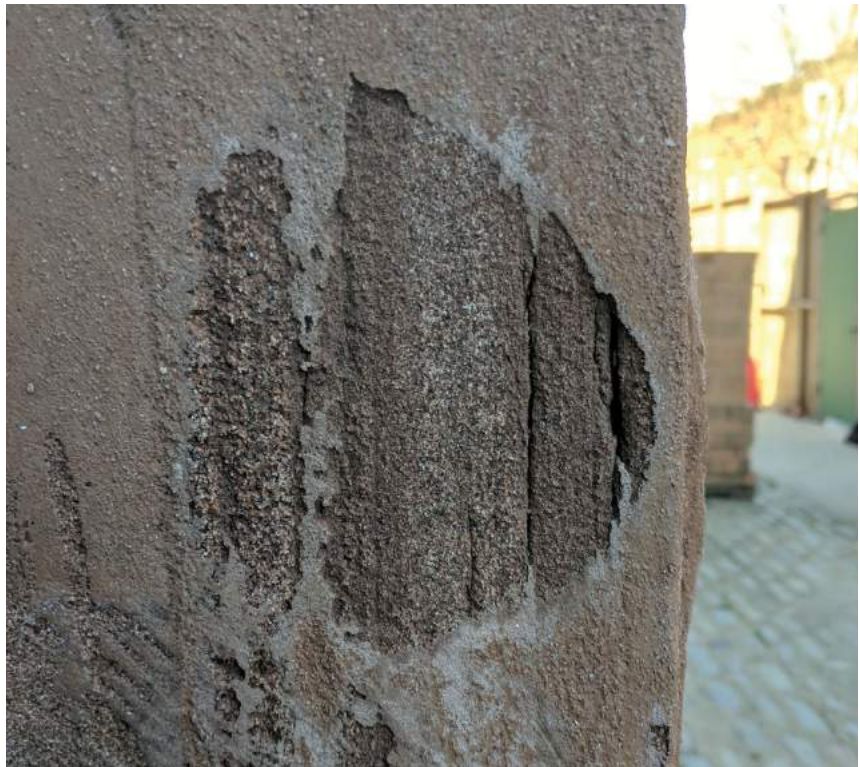
Example of a minor probe. A very small portion was carefully removed to determine the condition of the underlying material. This type of probe would not require a permit.
