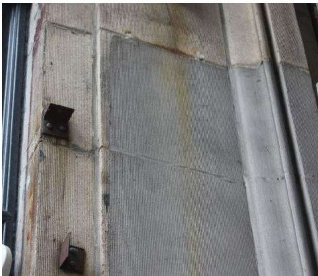
Example of inappropriate coating. In addition to being a poor color match, the coating extends over the mortar joints, sealing the masonry and mortar and restricting moisture transmission, which could accelerate deterioration.
