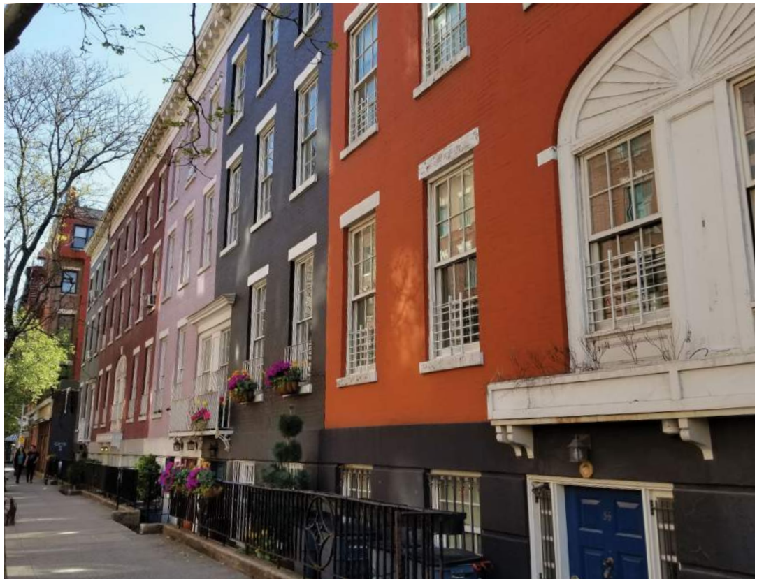
These rowhouses in the MacDougal-Sullivan Gardens Historic District were historically painted in a variety of colors.
