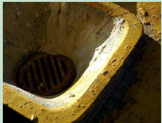
Drains and pipes.
