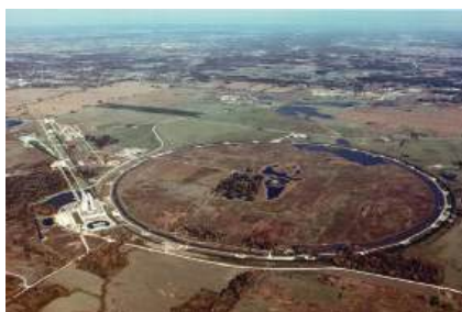
Figure 24.2.7 A Synchrotron An aerial photograph of what is currently the world's most powerful particle accelerator, the Tevatron at the Fermi National Accelerator Laboratory (Fermilab) in Illinois. The large tube characteristic of a synchrotron is 4 miles in circumference, contains 1000 superconducting magnets cooled by liquid helium, and can accelerate a beam of protons to almost the speed of light, giving them an energy greater than 1 TeV (teraelectronvolt = 10^3 GeV = 10^{12} eV) for collisions with other particles.
