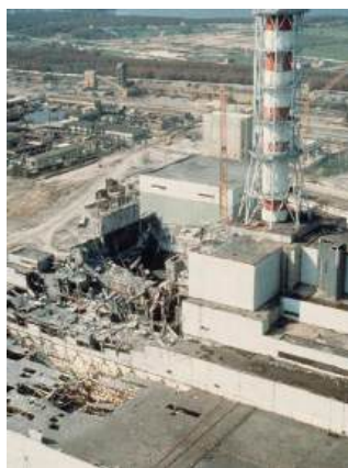
Figure 24.5.2 The Chernobyl Nuclear Power Plant In 1986, mechanical and operational failures during testing at the Chernobyl power plant in the USSR (now in the Ukraine) caused an uncontrolled nuclear chain reaction. The resulting fire destroyed much of the facility and severely damaged the core of the reactor, resulting in the release of large amounts of radiation that was spread over the surrounding area by the prevailing winds. The effects were devastating to the health of the population in the region and to the Soviet economy.
