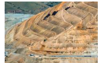
Figure 7.8 Construction Project in South America
