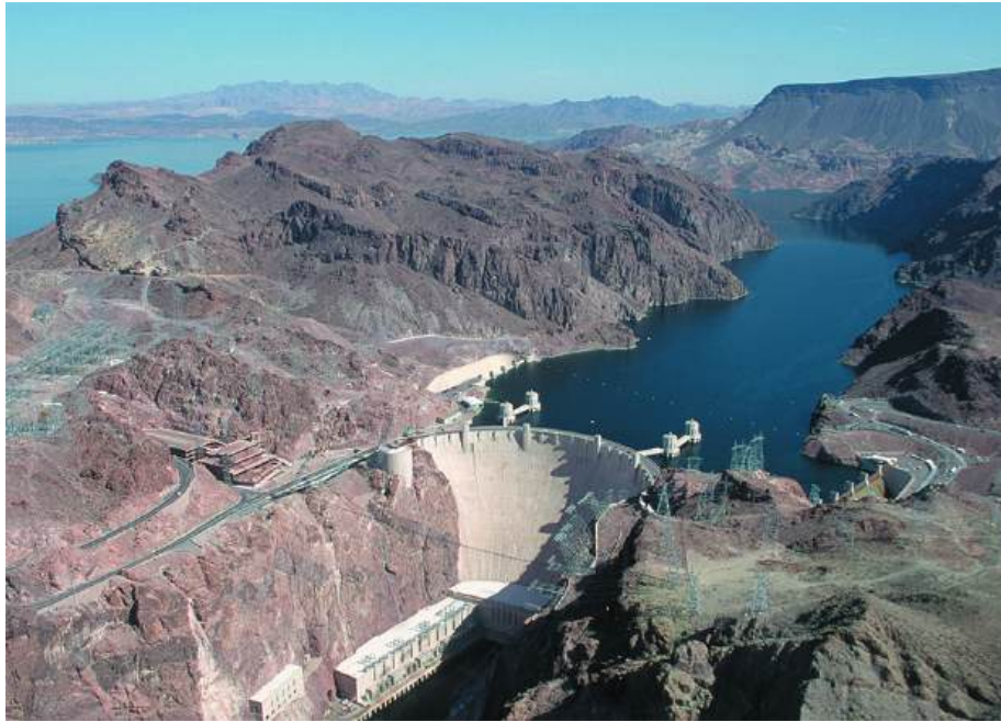
Figure 7.0.1: Hoover Dam is one of the United States' iconic landmarks, and provides irrigation and hydroelectric power for millions of people in the southwest United States. (credit: modification of work by Lynn Betts, Wikimedia).
