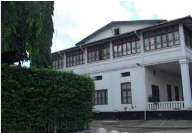
FIGURE 3.11-26 LARGE OPENINGS AND VERANDAS FOR NATURAL VENTILATION
