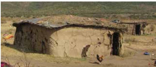
FIGURE 3.11-9 MASAI, KENYA: THE ENVELOPE IS MADE WITH COW DUNG AND ASH OVER A STRUCTURE IN WOOD AND THATCH
