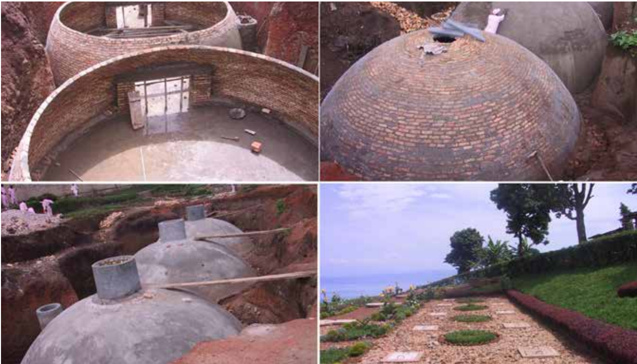
FIGURE 5.2-5 DIGESTERS CONSTRUCTION STAGES
