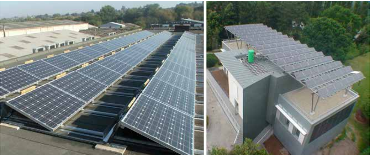
FIGURE 6.1-2 PV ON FLAT ROOF
