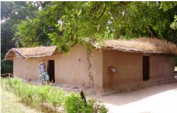
FIGURE. 3.11-1 HEHE TRADITIONAL HOUSE
