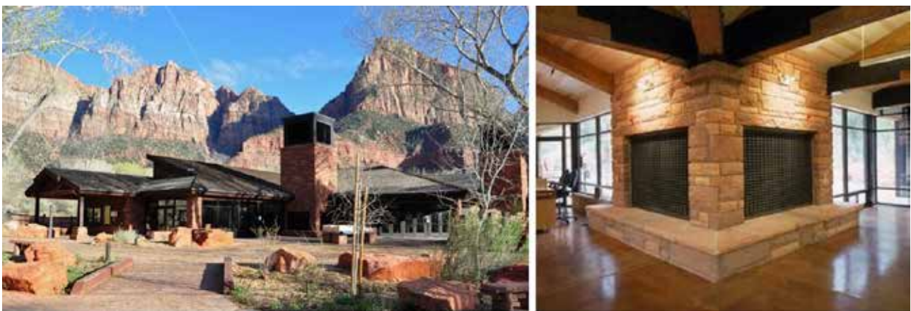
FIGURE 3.8-4 ZION NATIONAL PARK VISITOR CENTER (LEFT) AND COOLING TOWER OUTLET (RIGHT)
