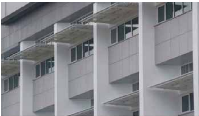
FIGURE 7.1-11 SHADING AND DAYLIGHTING FEATURES
