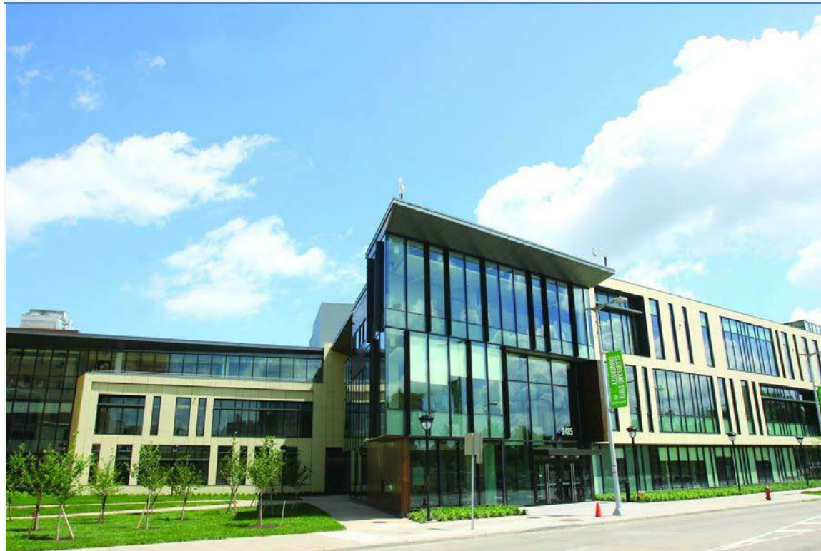
Figure 5.1 Outfitting a New Building
