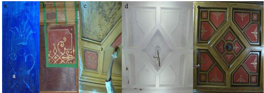
Figure 15. The show of the hidden decorative at the ceiling of one of the rooms of Sursoq Palace in Alexandria by discovering the original layers of decoration, which were hidden under new accumulated paints layers.
