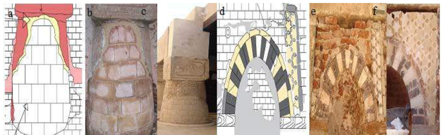
Figure 10. Multiple and variety methods for completion (a, b, c) completion of missing parts from sand stone in one of the columns of the Luxor Temple (d, e, f) completion of the missing composition elements of bricks, stone and wood in the mihrab of Abu Al Hagag mosque.
