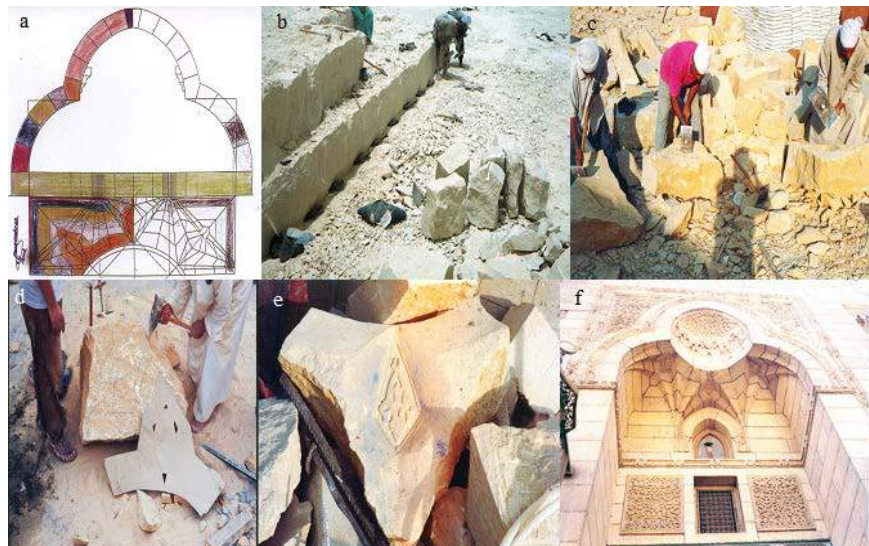
Figure 2. Evolution of the formation journey from the beginning of (a) the drawing & design; (b) the process of quarrying; (c) the process of refinement and primary sculpture; (d) the process of sculpting and removing the outside the design lines; (e) the process of finishing sculpture; (f) construction process and access to the simulated model of the original formation.
