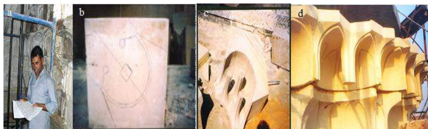
Figure 1. Restorer's tools for restoration formed elements; (a) read and understand, (b) drawings, (c) the process of sculpture and finishing, (d) construction.
