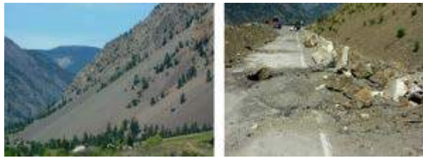
Figure 15.8 Left: A talus slope near Keremeos, B.C., formed by rock fall from the cliffs above. Right: The results of a rock fall onto a highway west of Keremeos in December 2014. [SE]
