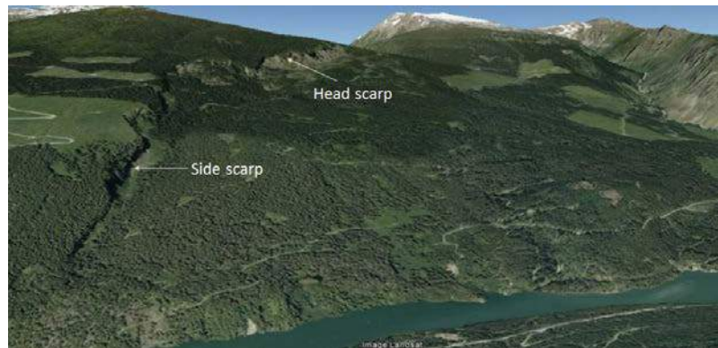
Figure 15.9 The Downie Slide, a sackung, on the shore of the Revelstoke Reservoir (above the Revelstoke Dam). The head scarp is visible at the top and a side-scarp along the left side. [from Google Earth]
