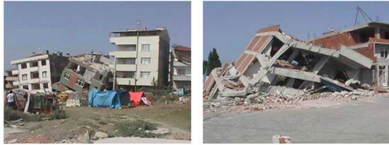
Figure 11.18 Buildings damaged by the 1999 earthquake in the Izmit area, Turkey. [from U.S. Geological Survey at: http://gallery.usgs.gov/sets/1999_Izmit_Turkey_Earthquake/thumb/_/1 ]
