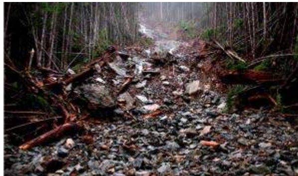
Figure 15.17 The lower part of debris flow within a steep stream channel near Buttle Lake, B.C., in November 2006. [SE]
