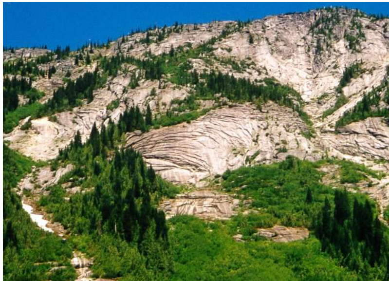
Figure 5.3 Exfoliation fractures in granitic rock exposed on the west side of the Coquihalla Highway north of Hope, B.C. [SE]
