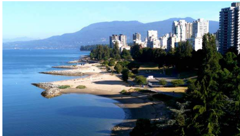
Figure 17.30 Photograph of the impact of breakwaters on beach development at Sunset Beach, Vancouver [by Isaac Earle, used with permission]
