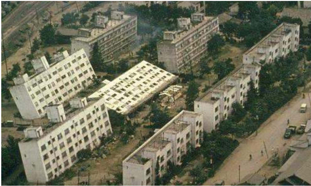
Figure 11.22 Collapsed apartment buildings in the Niigata area of Japan. The material beneath the buildings was liquefied to varying degrees by the 1964 earthquake. http://en.wikipedia.org/wiki/1964_Niigata_earthquake#/media/File:Liquefaction_at_Niigata.JPG
