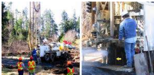
Figure 14.10 A water-well drilling rig in operation in the Cassidy area, near Nanaimo, B.C. In the photo on the right the well is being test-pumped with air pressure. The casing (yellow arrow) is about 40 cm in diameter. [SE]
