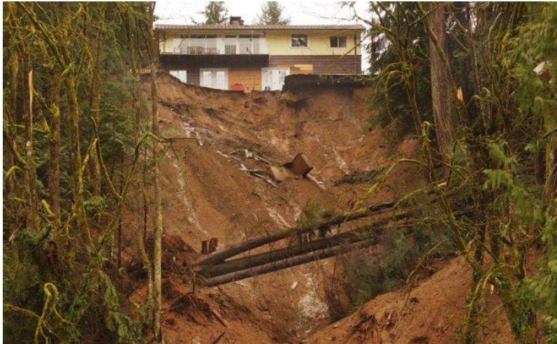
Figure 15.6 The debris flow in the Riverside Drive area of North Vancouver in January, 2005 happened during a rainy period, but was likely triggered by excess runoff related to the roads at the top of this slope and by landscape features, including a pool, in the area surrounding the house visible here. [The Province, used with permission]
