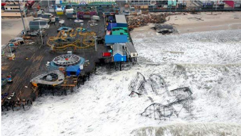
Figure 19.14 Damage to the Casino Pier, Seaside Heights, New Jersey, from Hurricane Sandy, November 2012 [ https://upload.wikimedia.org/wikipedia/commons/c/cb/Hurricane_Sandy_New_Jersey_Pier.jpg ]
