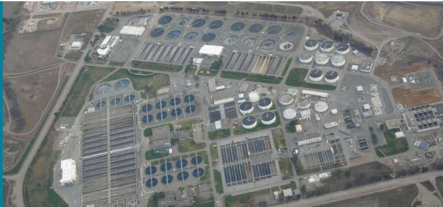
Figure 25.1 Sewage Treatment Plant (credit: "thekirbster"/flickr.com)
