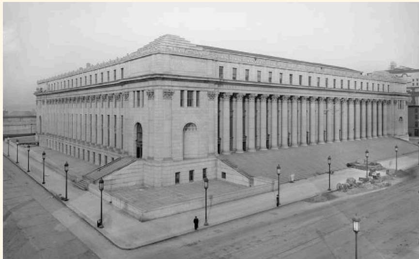
FIGURE 4.31 "Neither Snow nor Rain nor Heat nor Gloom of Night." The unofficial motto of the U.S. Postal Service, which once also described the Persian Empire's courier system, is inscribed on the face of this New York City building, over the colonnade. (credit: modification of work " Post Office, New York City (https://www.loc.gov/pictures/resource/det.4a24669/) " by Library of Congress Prints and Photographs Division/Library of Congress)
