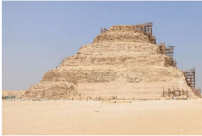
FIGURE 3.20 The Pyramid of Djoser. The Pyramid of Djoser, sometimes called the step pyramid, is composed of six stone mastabas set atop each other, each slightly smaller than the one below. Built by the architect Imhotep during the reign of Pharaoh Djoser, it is the earliest large stone building in Egypt. (credit: "Pyramid of Djoser (Step Pyramid)" by Jorge Láscar/Flickr, CC BY 2.0)
