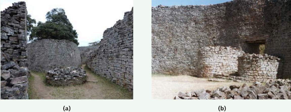
FIGURE 15.16 Great Zimbabwe Walls. (a) The Zimbabwean plateau features many impressive ancient structures constructed of drystone, that is, walls that do not rely on mortar. (b) The interior of the Great Enclosure can be seen in this photo of the entrance to the main enclosure. (credit a: modification of work “Great Zimbabwe 8” by Mike/Wikimedia Commons, CC BY 2.0; credit b: modification of work “Great Zimbabwe, Main enclosure entrance” by “damien_farrell”/Flickr, CC BY 2.0)
