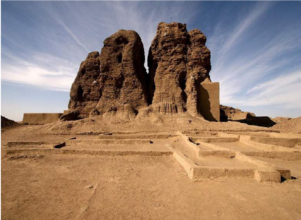
FIGURE 9.15 The Western Deffufa. Kerma’s Western Deffufa is one of three such massive temples known to exist. It is fifty-nine feet tall, and its complex extends over fifteen thousand square feet. (credit: “Western Deffufa – Kerma” by Walter Callens/Wikimedia Commons, CC BY 2.0)
