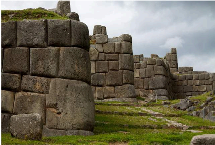
FIGURE 8.33 Inca Stonework at Sacsayhuamán. While many of the Inca-built parts of Cuzco were destroyed in later centuries, the sixteenth-century site of Sacsayhuamán nearby preserves its ancient walls of stones, so skillfully hewn as to fit together tightly without mortar. (credit: “Peru - Cusco Sacred Valley & Incan Ruins 005 – Sacsaywamán” by McKay Savage/Flickr, CC BY 2.0)
