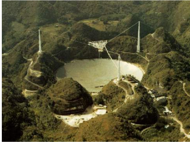
Figure 6.22 Largest Radio and Radar Dish. The Arecibo Observatory in Puerto Rico was the largest and most powerful astronomical radar facility in the world and was often featured in films. In November 2020 it collapsed, damaging the 300-meter diameter “dish” and destroying the radar transmitter and receiver. (credit: National Astronomy and Ionosphere Center, Cornell U., NSF)
