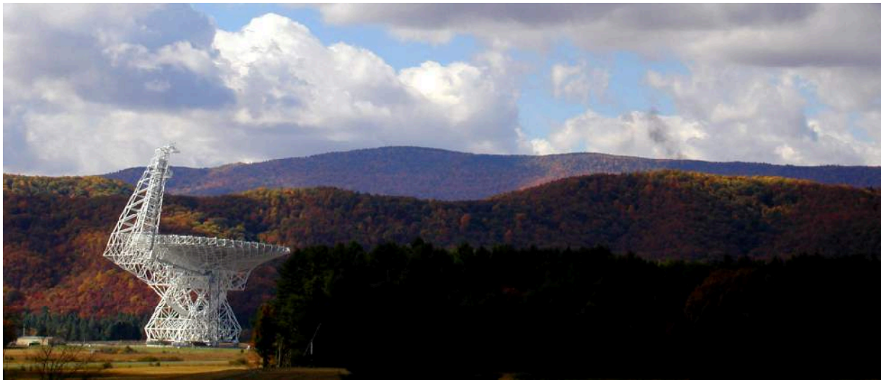
Figure 6.19 Robert C. Byrd Green Bank Telescope. This fully steerable radio telescope in West Virginia went into operation in August 2000. Its dish is about 100 meters across. (credit: modification of work by "b3nscott"/Flickr)
