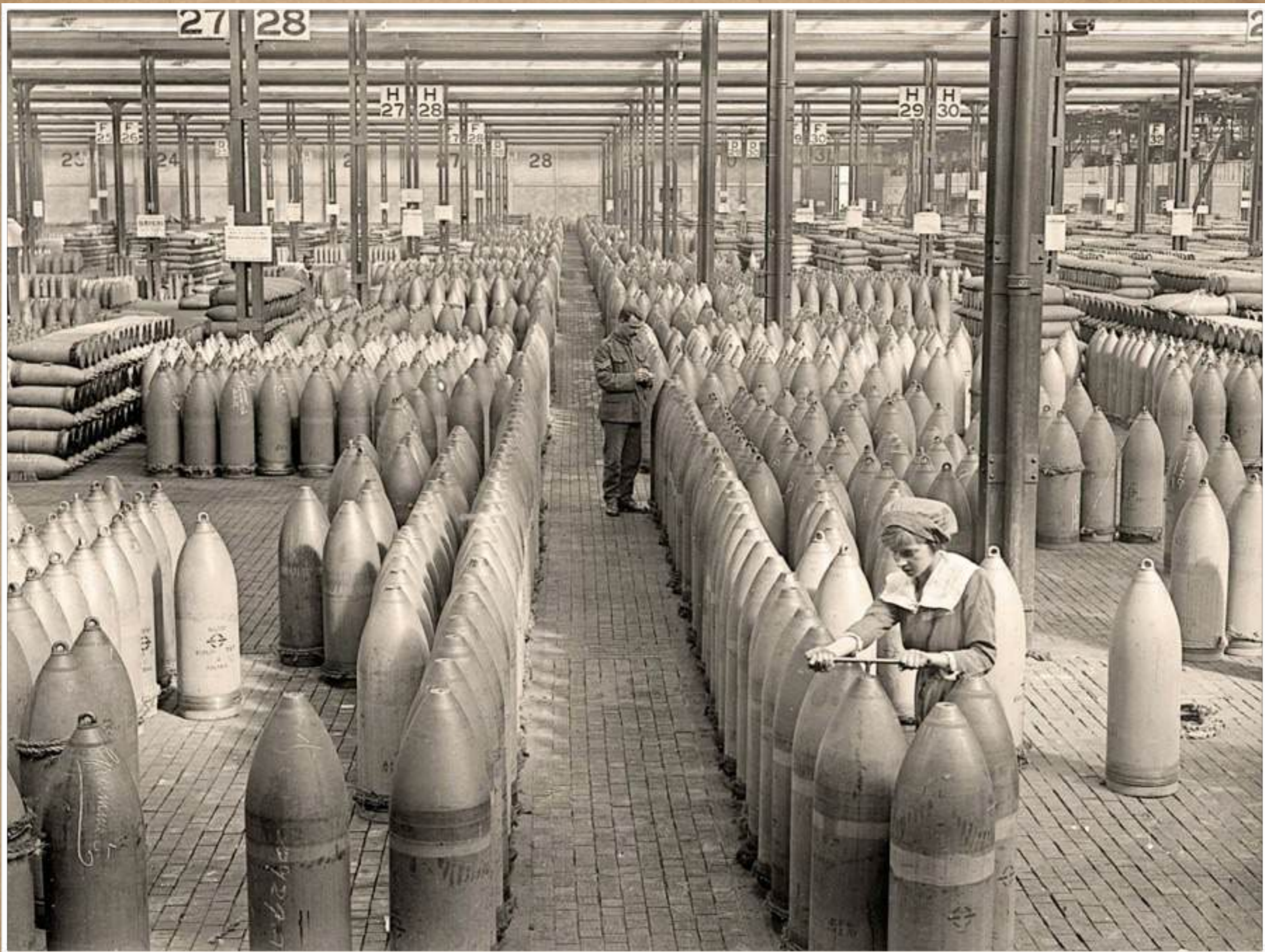
Workers at Chilwell factory in Nottinghamshire checking and tightening shells. IWM (Q 30041)
