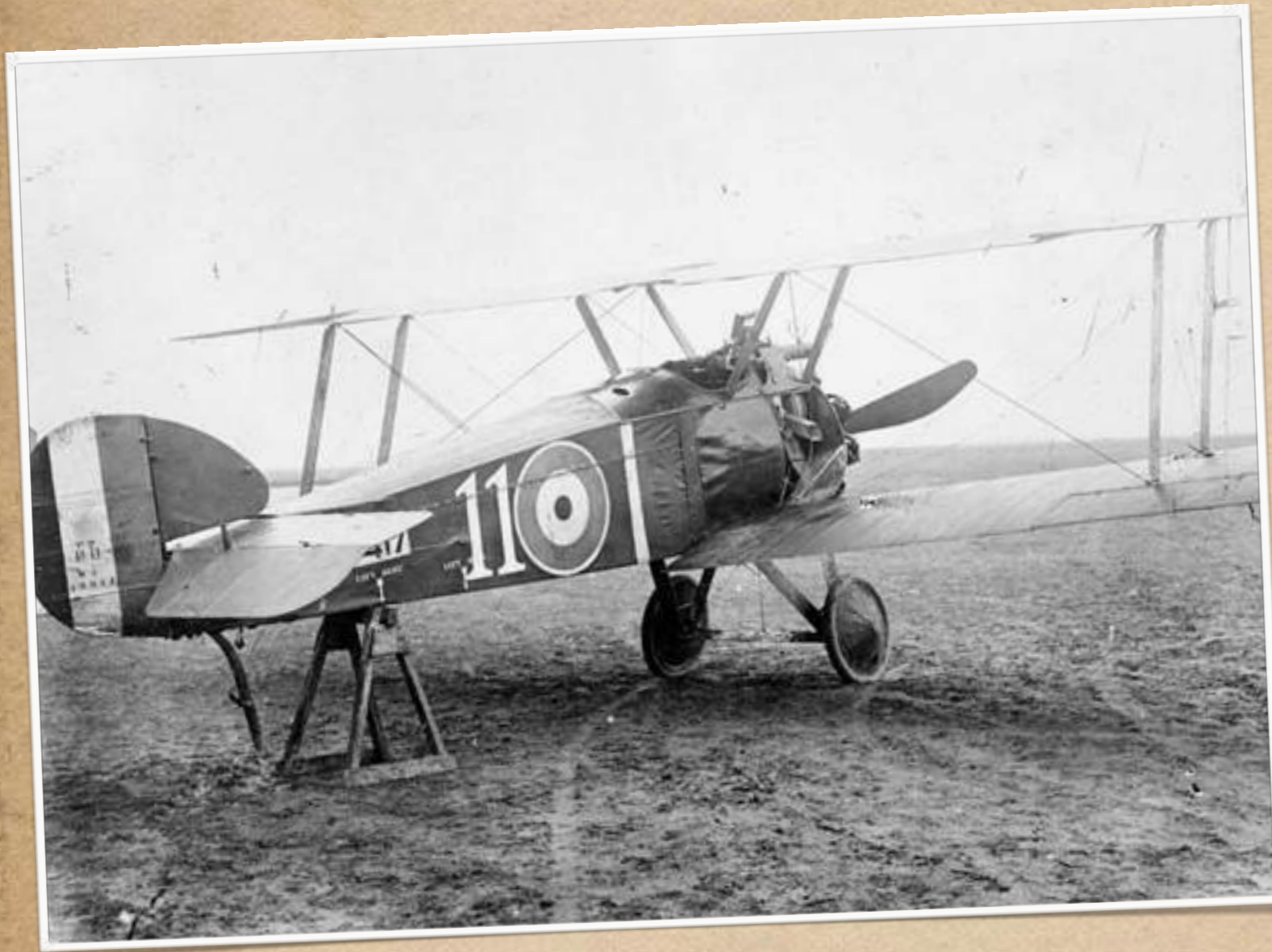
The Sopwith Camel (above) had a maximum speed of 115mph and was named after the hump-shaped protective covering over its machine guns. IWM (Q 073399)
