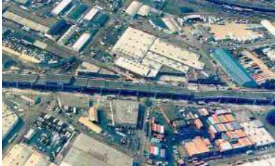
1 / The collapsed section of the Nimitz Freeway
