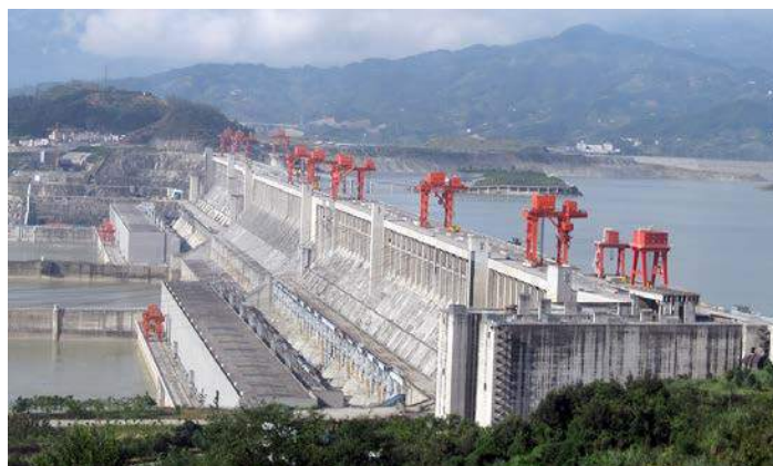
Figure 11.5 Three Gorges Dam in central China. When completed in 2008, this became the world's largest hydroelectric plant, generating power equivalent to that generated by 22 average-sized nuclear power plants. The concrete dam is 181 \text{ m} high and 2.3 \text{ km} across. The reservoir made by this dam is 660 \text{ km} long. Over 1 million people were displaced by the creation of the reservoir. (credit: Le Grand Portage)
