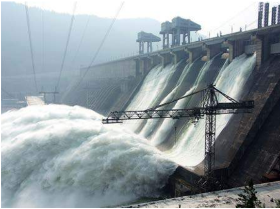
Figure 7.38 Hydroelectric facility (credit: Denis Belevich, Wikimedia Commons)
