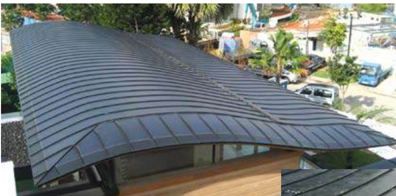
Figure A.4.2. Lightweight, flexible laminates follow the curved roof
