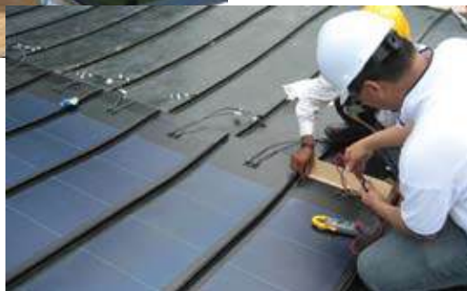
Figure A.4.3. Testing the Uni-Solar laminates during installation
