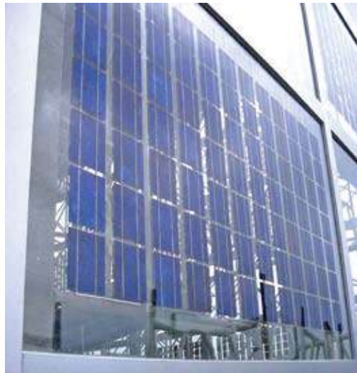
Figure 15. BIPV modules integrated into a façade
