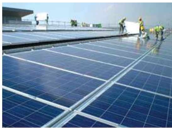
Figure A.6.3. Installing the REC modules
