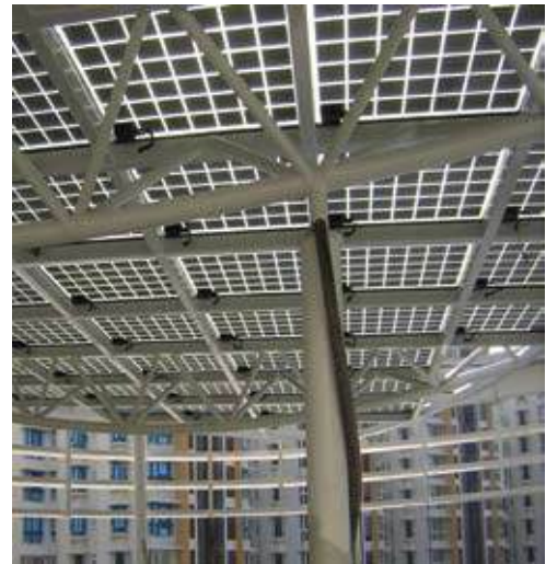
Figure 16. BIPV modules integrated into a skylight canopy
