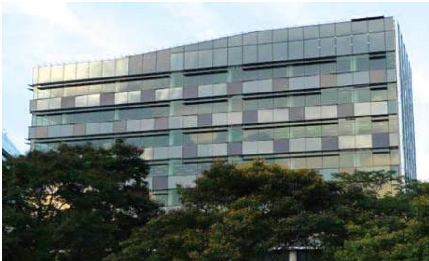
Figure A.8.1. 6kWp BIPV façade on Tower 2
