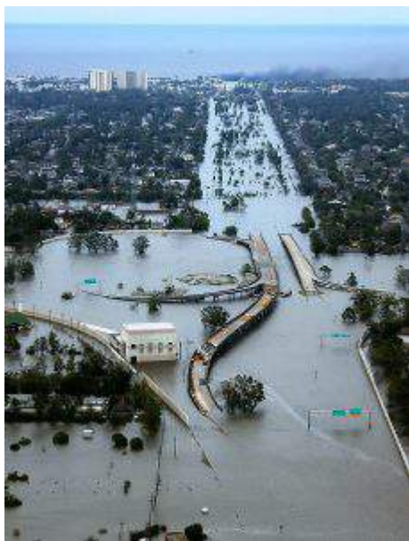
Figure 10.13: In 2005, boundaries between organizations hampered rescue efforts following Hurricane Katrina.
