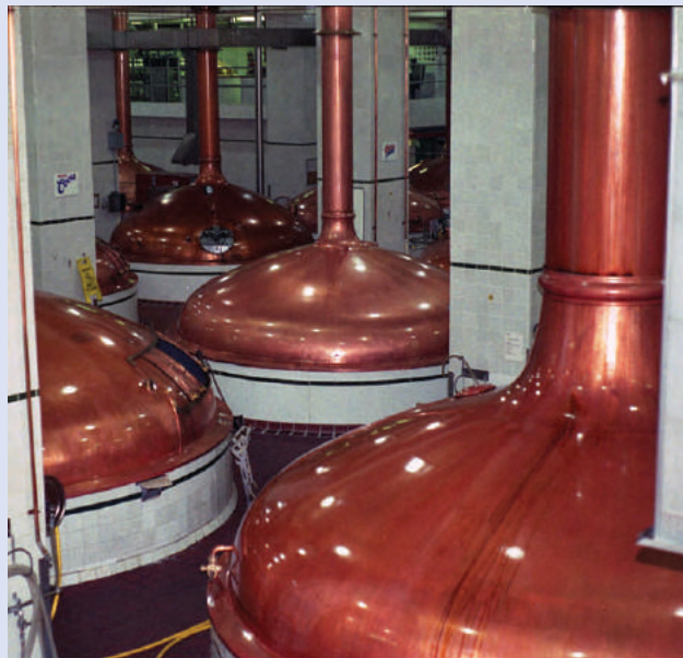
Figure 3.13 An oxide of carbon is removed from these fermentation tanks through the large copper pipes at the top. (credit: "Dual Freq"/Wikimedia Commons)
