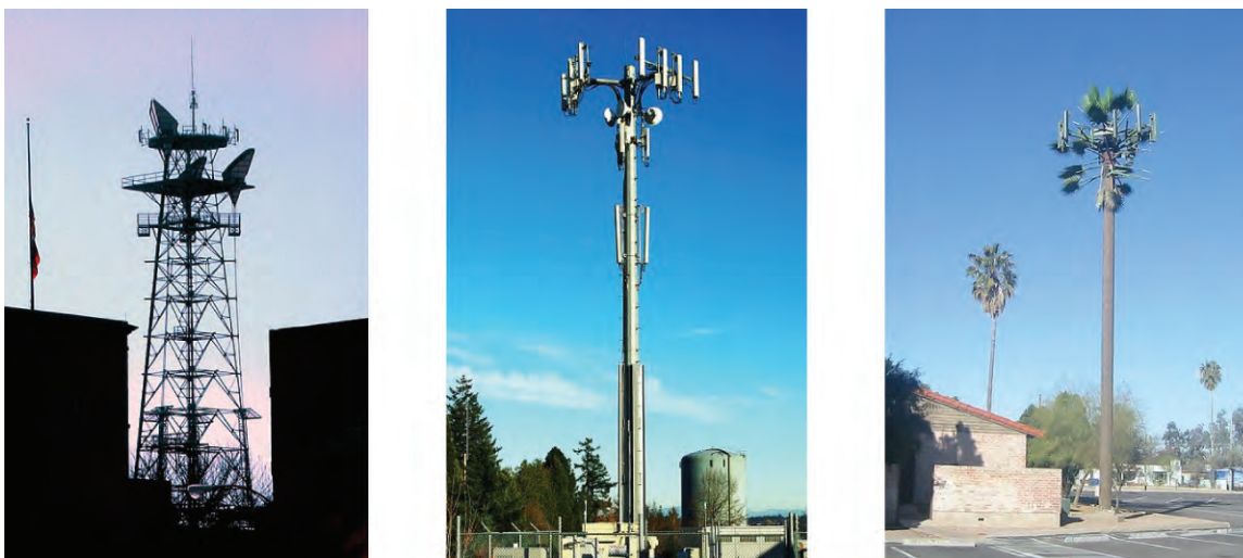
Figure 6.4 Radio and cell towers are typically used to transmit long-wavelength electromagnetic radiation. Increasingly, cell towers are designed to blend in with the landscape, as with the Tucson, Arizona, cell tower (right) disguised as a palm tree. (credit left: modification of work by Sir Mildred Pierce; credit middle: modification of work by M.O. Stevens)
