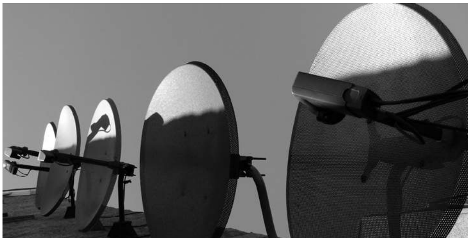
Figure 1 An array of satellite dishes. (credit: Matthew Colvin de Valle, Flickr)
