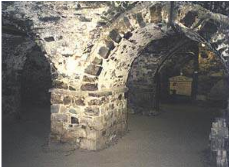
Photograph 1.1 - Foundations for a Medieval Era Cathedral
