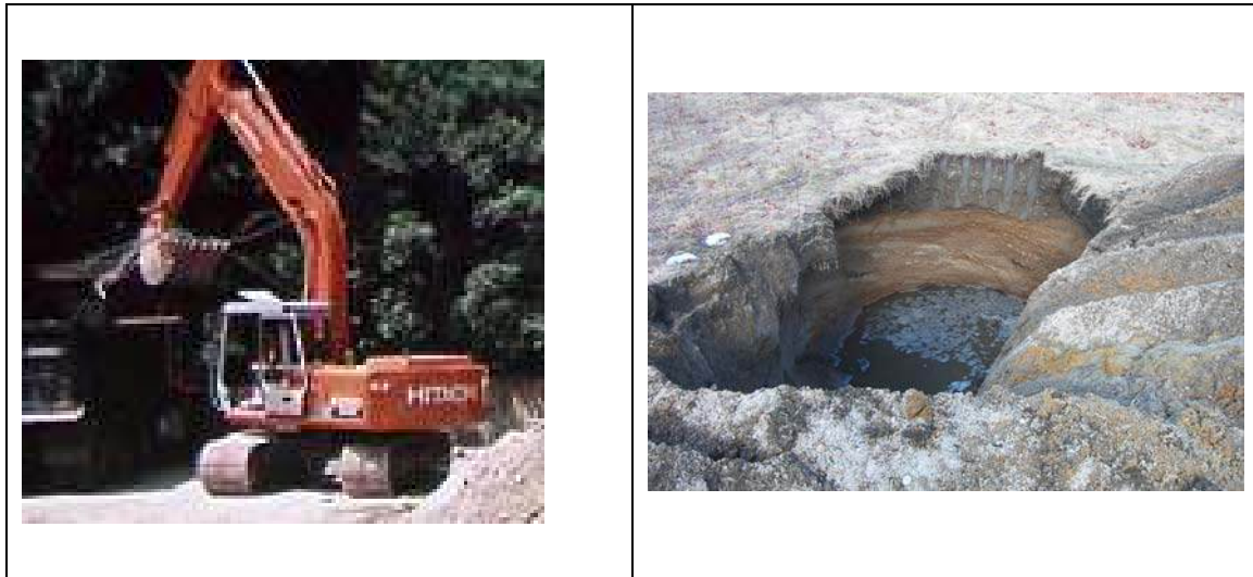
Photograph 2.1 – Test Pit Excavation
