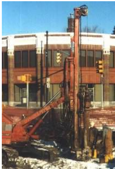
Photograph 8.1 - Drilling to Install a Small Diameter Grouted Pile
