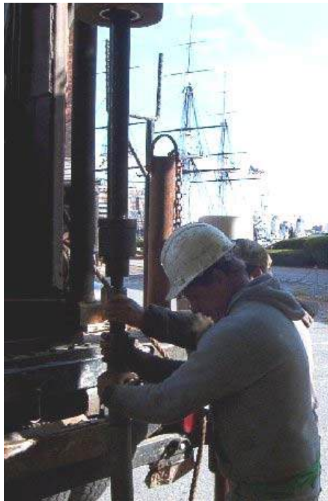
Photograph 2.2 – Standard Penetration Test
