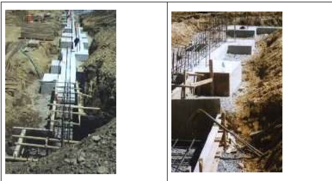
Photograph 4.1 – Shallow Spread Footings
