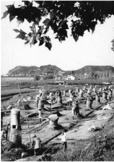
Backyard furnaces in China during the Great Leap Forward era produced very poor steel and a lot of pollution.
