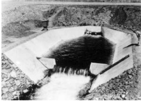
Figure 7-9 -- Cipolletti weir with a well-type head-measuring station.
