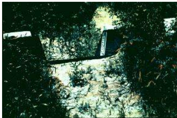
Figure 5-7 -- Sediment deposits in weir pool.
