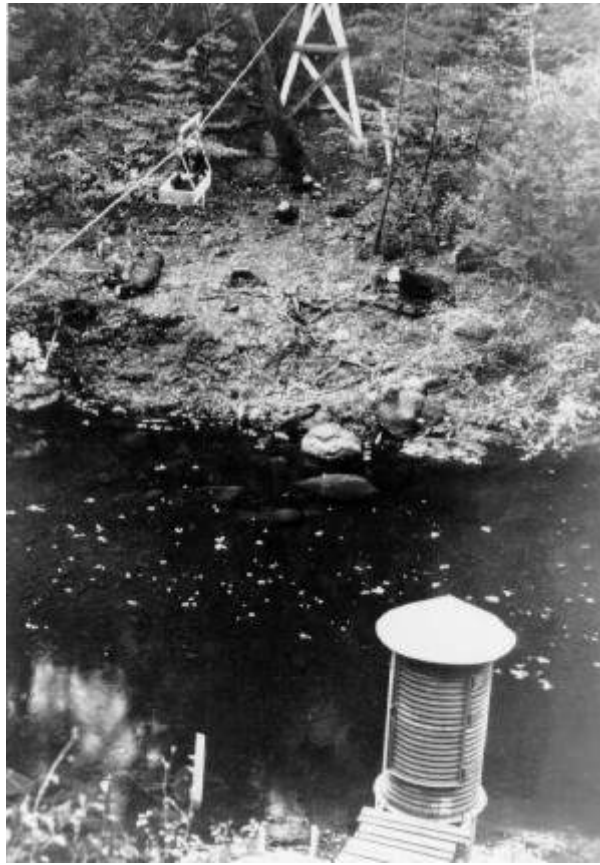
Figure 6-11 -- Current-meter gaging station with cable car, corrugated steel shelter house, and stilling well.
