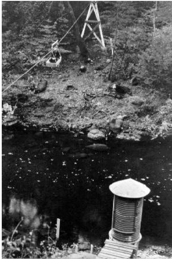
Figure 10-3 -- Current-meter gaging station with cable car, corrugated steel shelter house, and stilling well.
