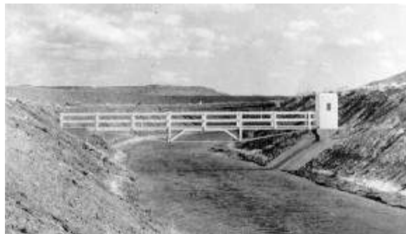
Figure 10-1 -- Current-meter station on a canal, viewed from upstream. Current-meter measurements are taken from the bridge, and the sheltered stilling well houses an automatic water-stage recorder.
