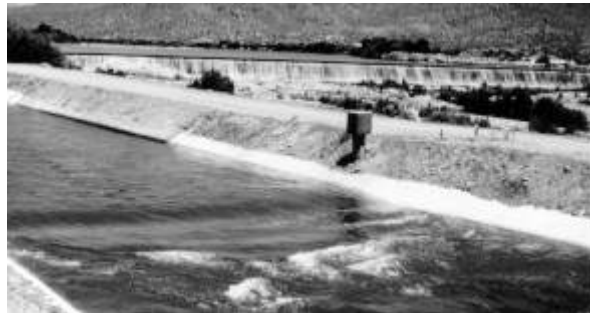
(b) The long-throated flume (broad-crested weir) with approximately 1,200 ft 3 /s.
