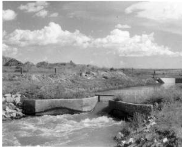
Figure 8-2 -- Four-foot, short-form Parshall flume, discharging 62 \text{ ft}^3/\text{s} under free-flow conditions. Scour Protection is needed for this much drop.
