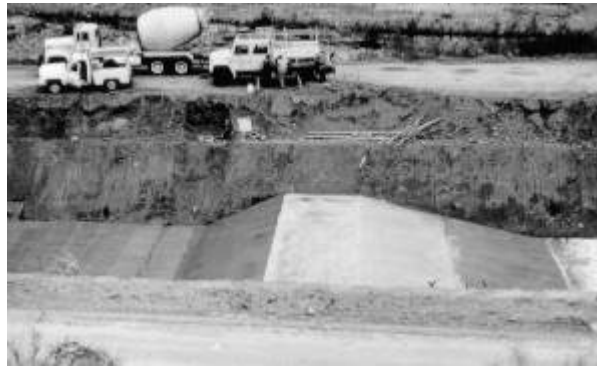
(a) Long-throated flume (broad-crested weir) under construction.
