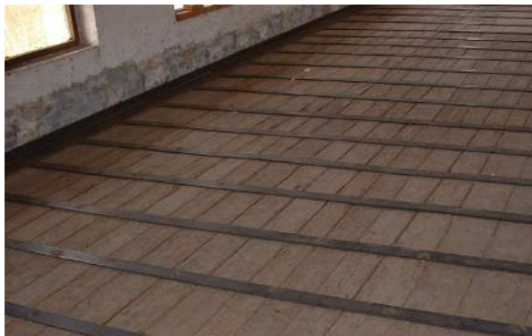
Figure 92 – Example of strengthening in bending of beams, by connecting steel strips to the compression zone.
