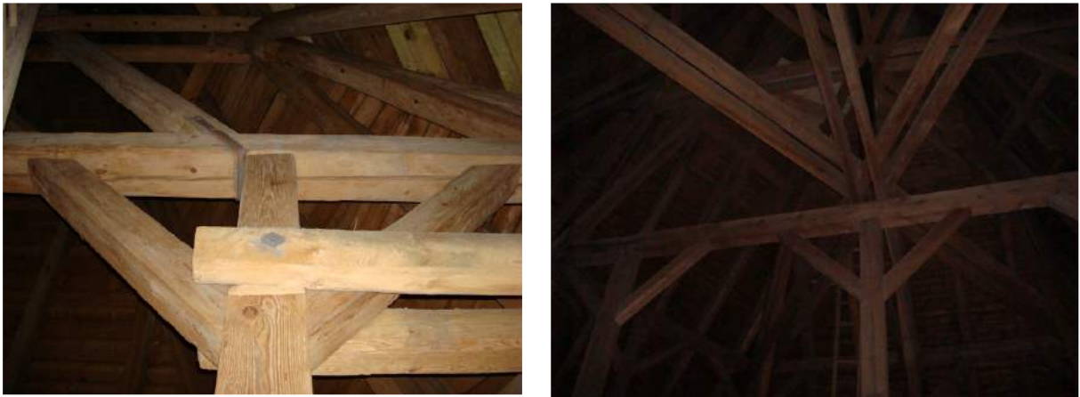
Figure 69 – Addition of timber bracing members (Kutna Hora Cathedral)
