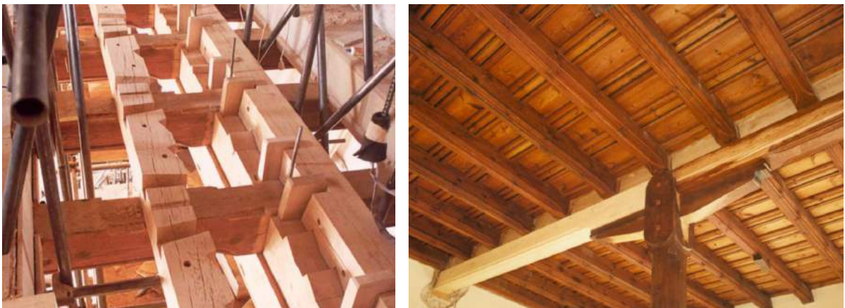
Figure 66 – .Carpentry based restoration of Karlštejn Castle timber floors.
