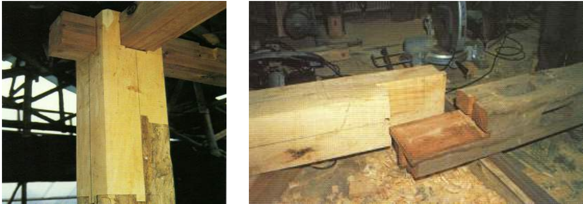
Figure 54 – Examples of timber prosthesis using traditional timber carpentry techniques (Japan).
