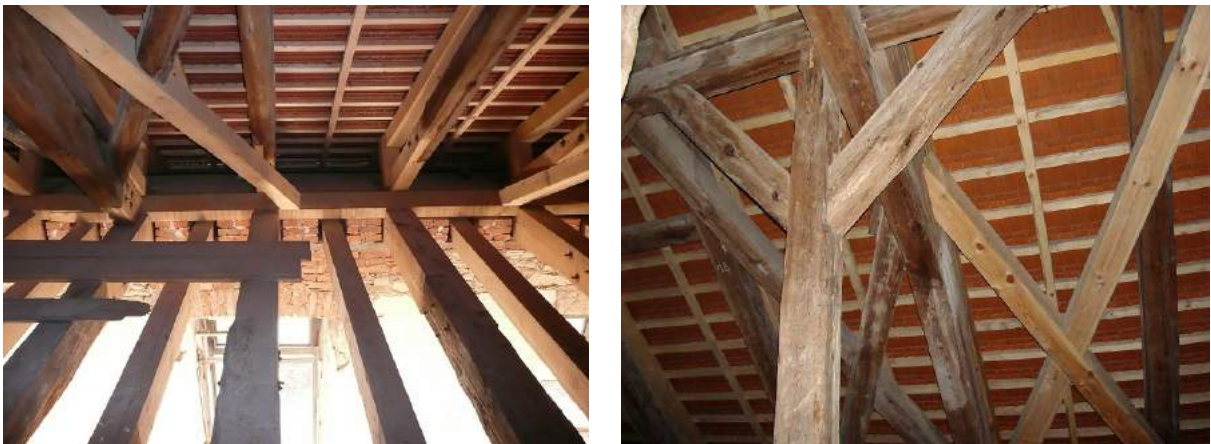
Figure 67 – Substitution of elements on Buštehrad Castle timber roof.
