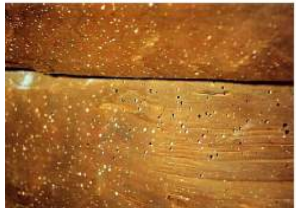
Figure 20 – Common furniture beetle bore holes.
