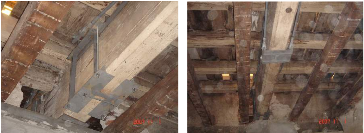
Figure 101 – Post-stressing of a beam.
