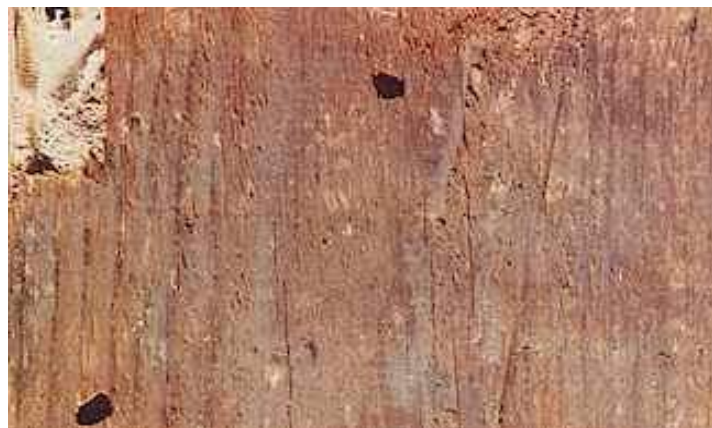
Figure 22 – House longhorn beetle bore holes
