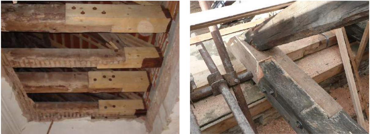
Figure 72 – Example of prosthesis with steel bolts as connectors (Buštehrad Castle).
