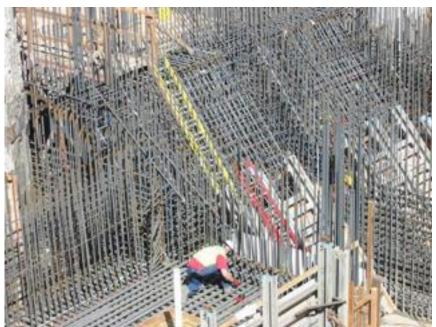
Rebar being set in place for the foundation of a sewage treatment plant pump station. Source: Wikipedia and licensed through Creative Commons.
