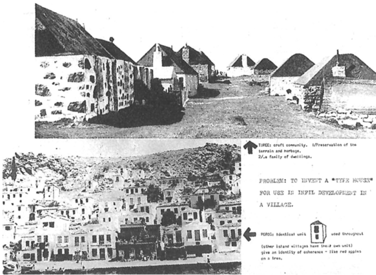
Figure 9.9. Alison and Peter Smithson, photograph of Poros island in Greece showing the aggregation of units. Detail of CIAM grille entitled “Housing Appropriate to the Valley Section” presented at the 10 th CIAM.
