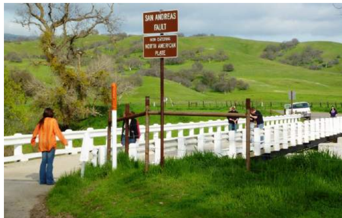
Figure 10.25 The San Andreas Fault at Parkfield in central California. The person with the orange shirt is standing on the Pacific Plate and the person at the far side of the bridge is on the North American Plate. The bridge is designed to slide on its foundation. [SE]
