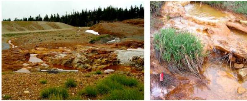
Figure 5.11 Exposed oxidizing and acid generating rocks and mine waste at the abandoned Mt. Washington Mine, B.C. (left), and an example of acid drainage downstream from the mine site (right). [SE]
