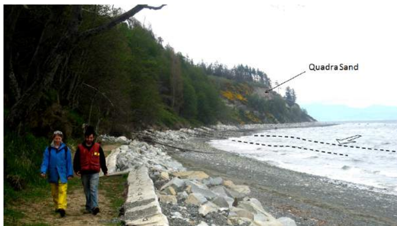
Figure 17.19 The Quadra Sand cliff at Comox, and the extensive concrete and rip-rap barrier that has been constructed to reduce erosion. Note that the waves (dashed lines) are approaching the shore at an angle, contributing to the longshore current. [SE]
