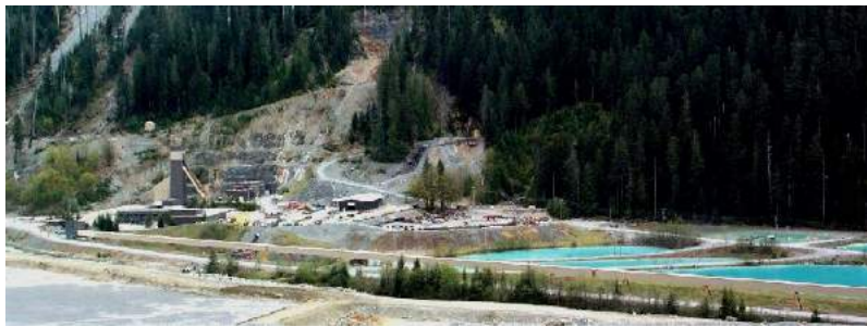
Figure 20.13 The tailings pond (lower left) at Myra Falls Mine with settling ponds (right) for processing water from the concentrator. [SE]
