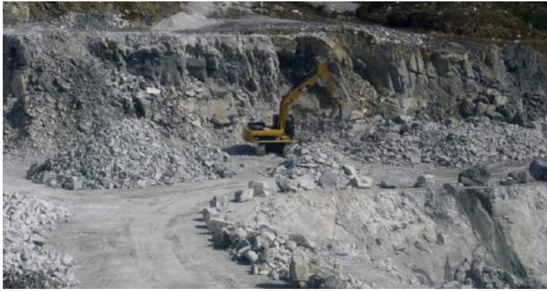
Figure 20.16 Triassic Quatsino Formation limestone being quarried on Texada Island, B.C. [SE]
