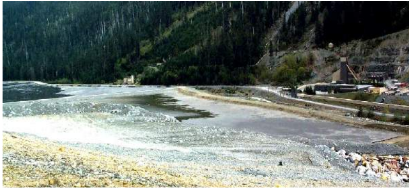
Figure 20.12 The tailings pond at the Myra Falls Mine on Vancouver Island. The dry rock in the middle of the image is waste rock. The structure on the right is the headframe for the mine shaft. Myra Creek flows between the tailings pond and the headframe. [SE]
