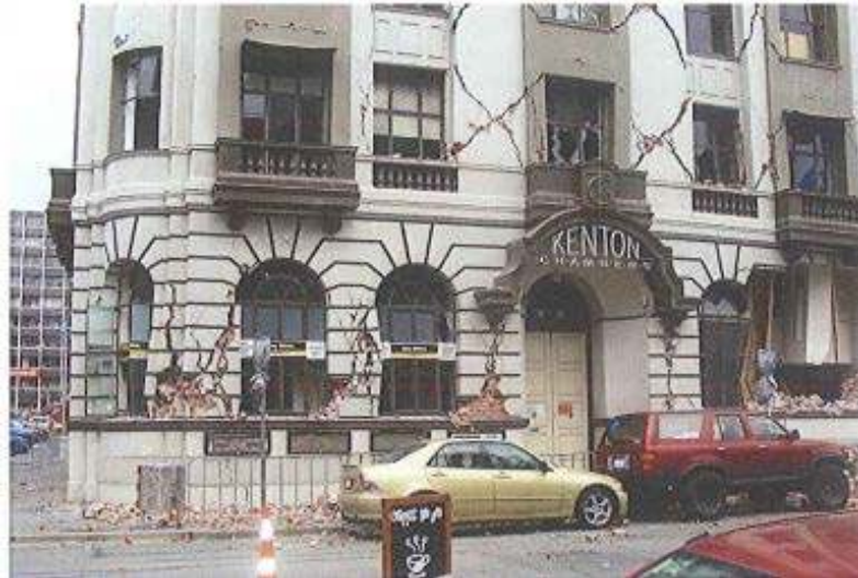
(a) Diagonal tension cracks to a brick pier. Note splitting of bricks (Dizhur)
