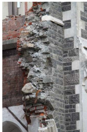
(b) Stone facing and brickwork backing
