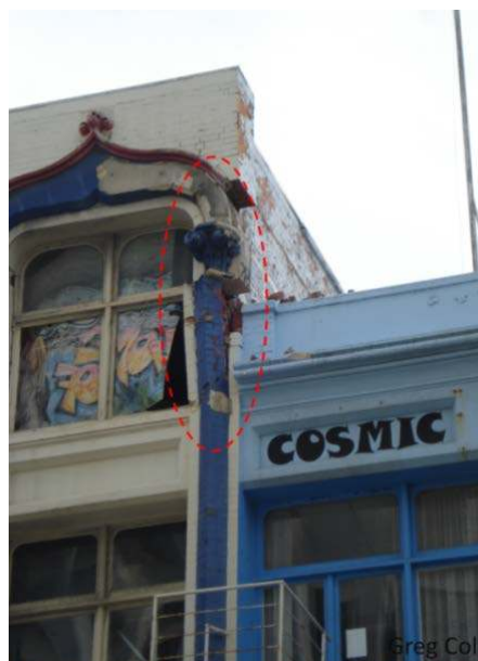
Figure C8.49: Pounding failure (Cole)
