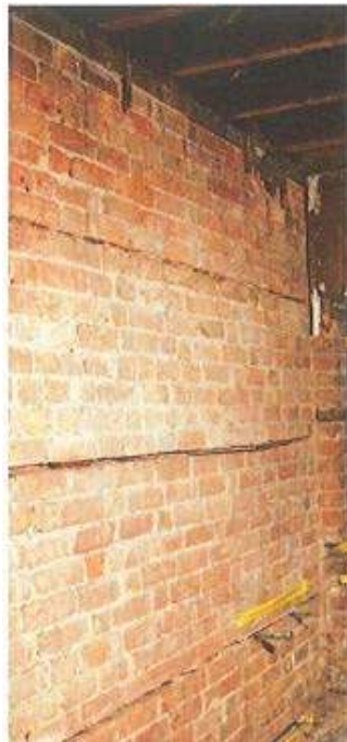
Figure C8.19: 12 mm timber built into every eighth course for fixing linings
