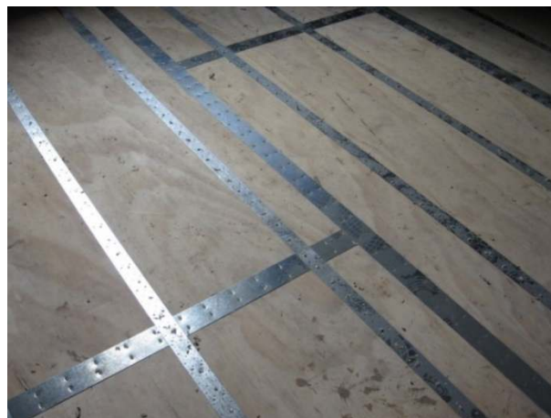
Figure C8.25: New plywood diaphragm (Holmes Consulting Group)
