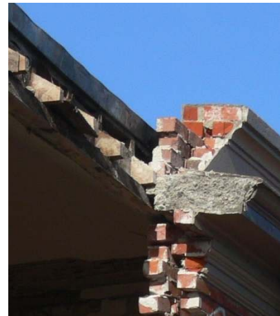
(b) Roof seating arrangement and parapet wall (Dymtro Dizhur)
