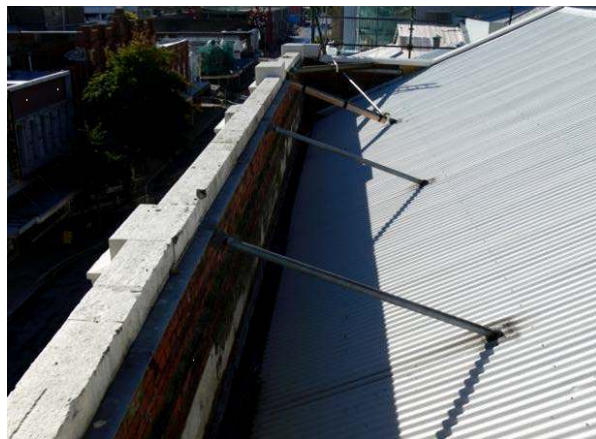
Figure C8.27: Parapet bracing. Note a lack of vertical tie-up of the parapet. (Dizhur)
