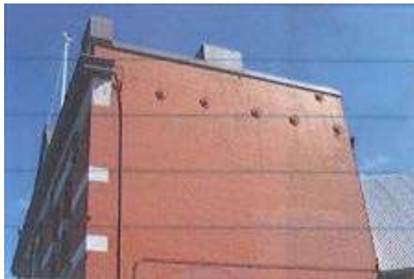
(a) Post-September 2010 event – minor visible damage
