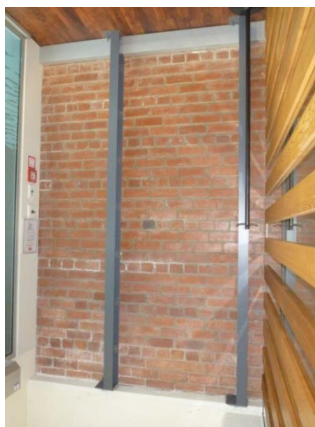
Figure C8.23: Bracing of wall against face load (Dunning Thornton)
