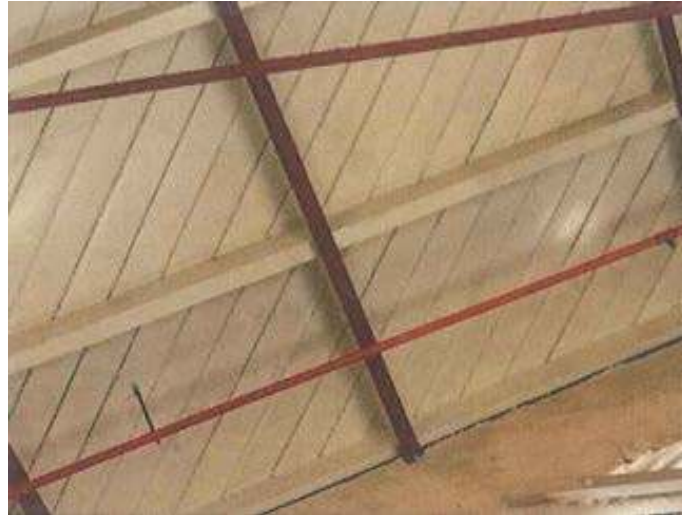
Figure C8.13: Typical timber diaphragms – diagonal sarking
