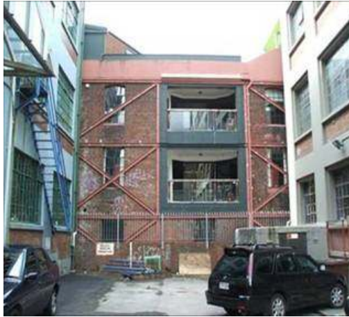
(a) Concentric steel frame (Beca)
