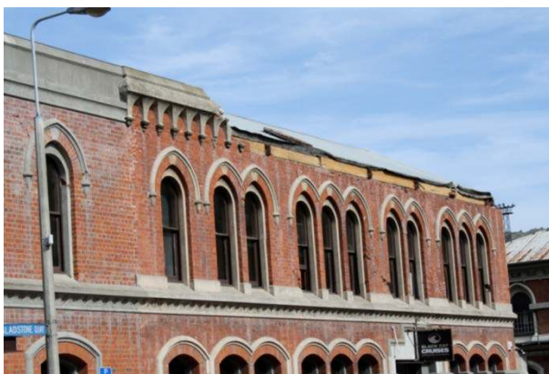
(a) Out-of-plane instability of parapet (Beca)
