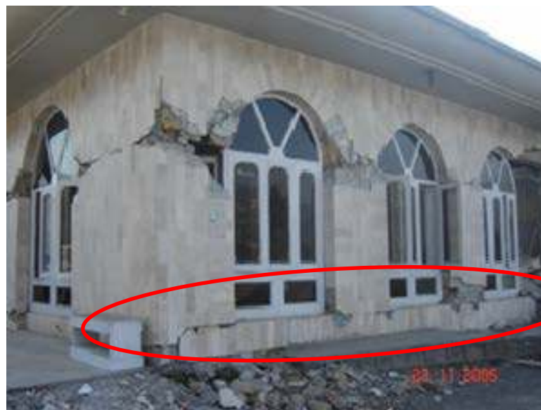
Figure C8.43: Rocking and delamination of bricks of a one-storey unreinforced brick masonry building with reinforced concrete roof slab (Bothara and Hıçılmaz, 2008)
