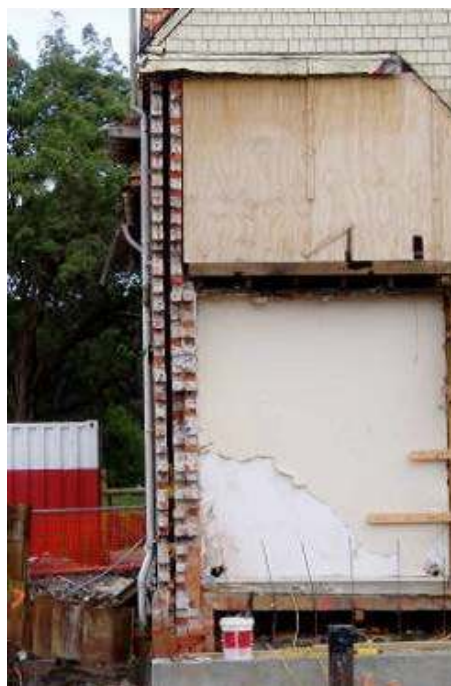
Figure C8.4: Change in cross section of brick wall (Holmes Consulting Group)
