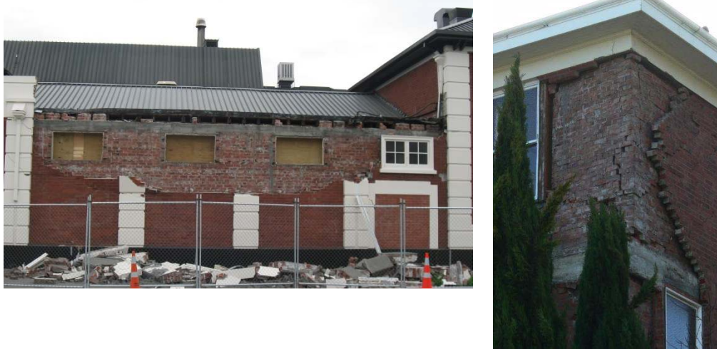
Figure C8.41: Failure of URM cavity walls (Dizhur)
