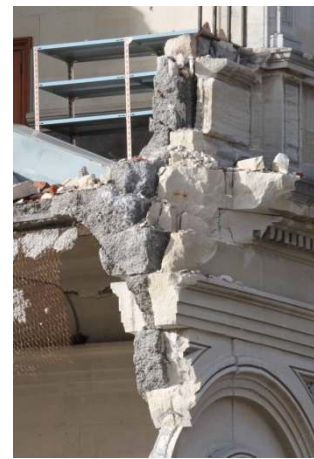
(c) Stone facing and concrete core
