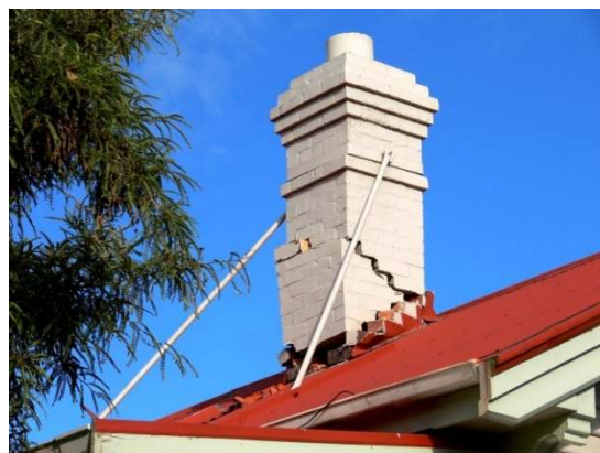
(b) Chimney at onset of falling (Dizhur)
