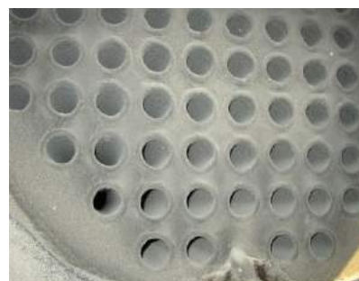
Figure 4-19: Fire-tube boiler (opened) [87]
