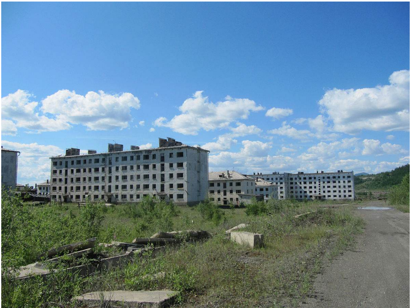
Figure 3.15: Abandoned Apartment Buildings in Kadykchan, Russia (© Laika ac, Wikimedia Commons, CC BY-SA 2.0)
