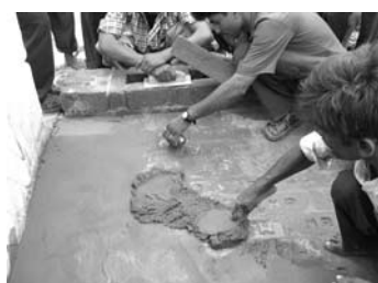
Placing the cement mortar
