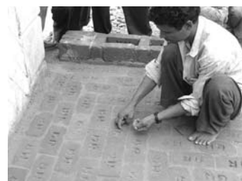
Cleaning the frog of the brick from wet sand for better binding
