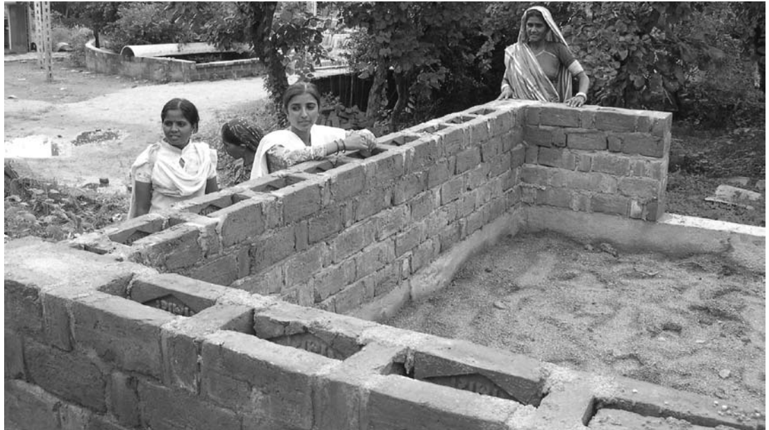
Ongoing brick wall (Rat Trap Bond) construction
