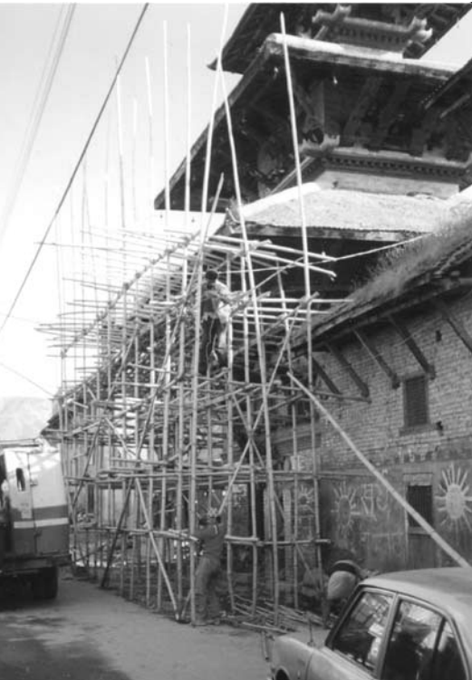
Scaffolding not properly protected from vehicles, workers at increased risk of serious accident
