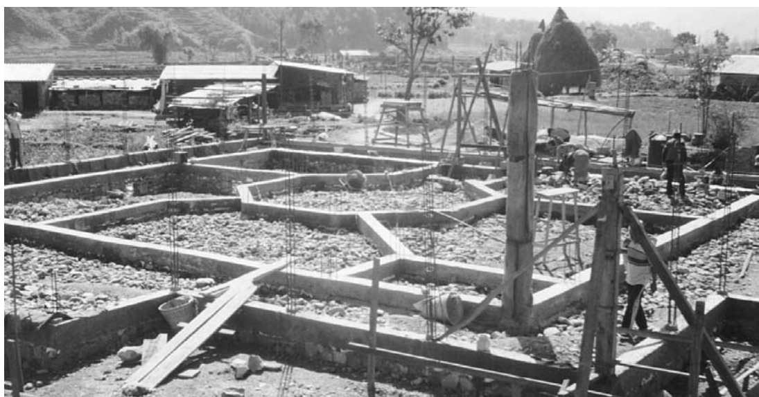
Completed plinth beam of a building
