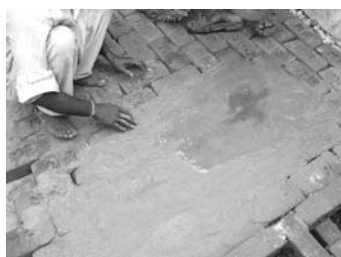
Filling the brick joints with wet sand
