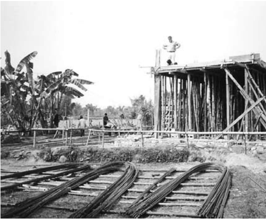
Steel bars properly stored at construction site.
