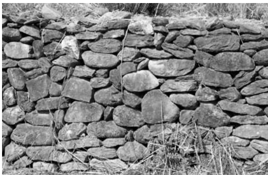
All size bolder stone try masonry wall
