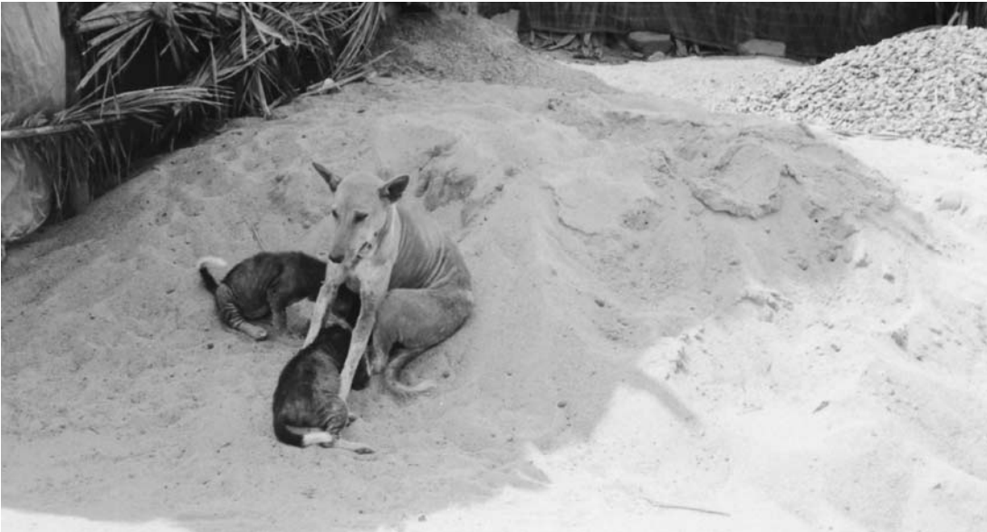
Dogs will contaminate concrete raw material, therefore proper protection is required
