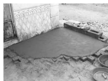
Brick bat floor example completed
