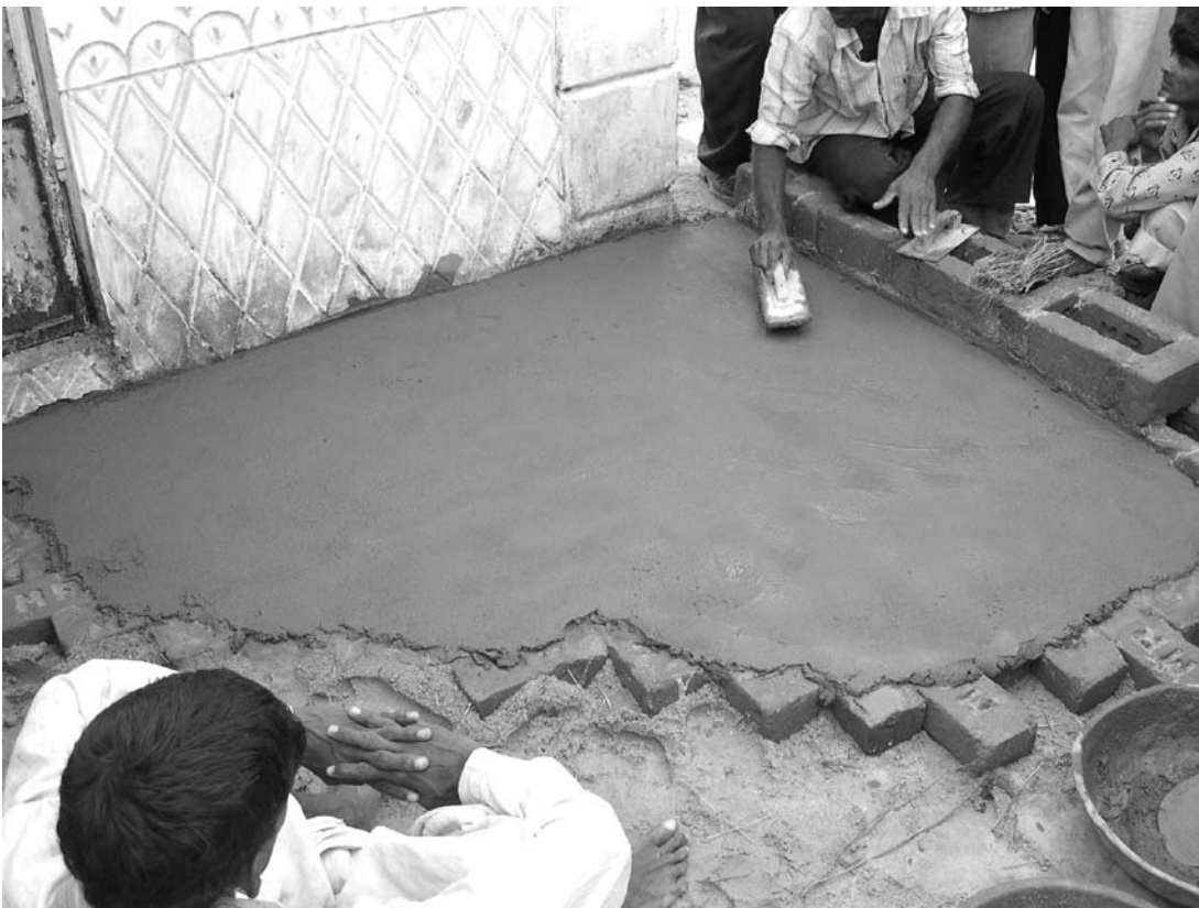
Floor construction section, levelling sand, brick layer, cement cover and finishing work
