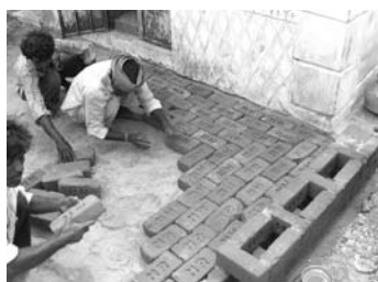
Laying bricks into a bed of sand
