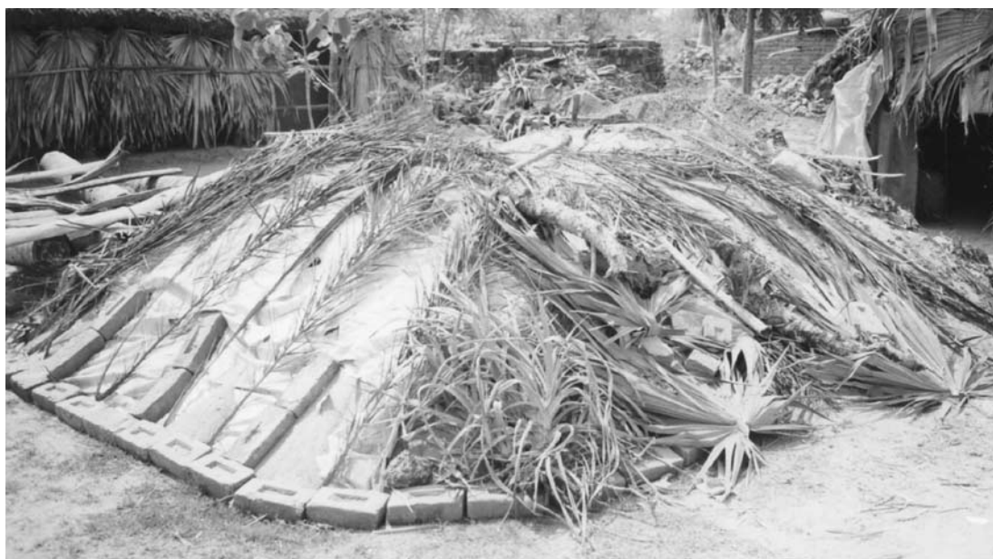
Sand deposit properly covered and protected from being contaminated
