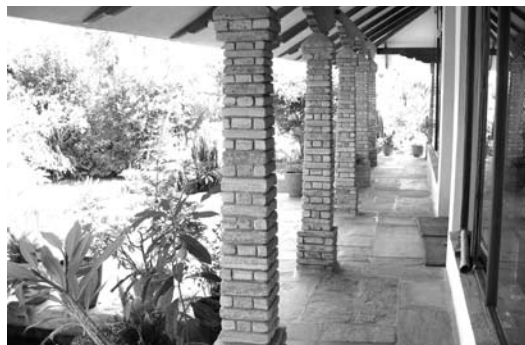
Sized stone pillar construction
