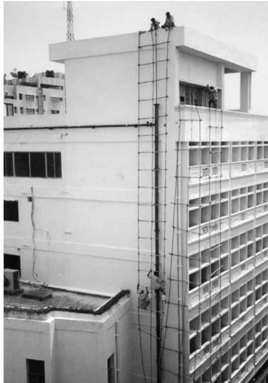
No proper working platform for wall painting made, workers at increased risk of serious accident
