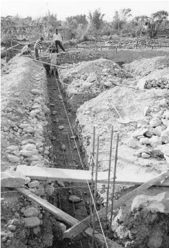
Steel reinforcement placing in foundation excavation
