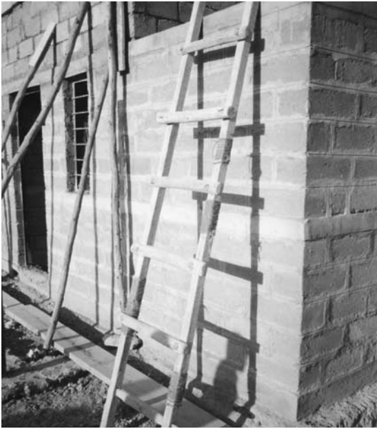
Continuous sill (direct below window) and lintel (direct above window)
