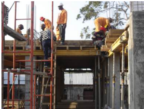
Figure 1.2.1: A building being constructed
