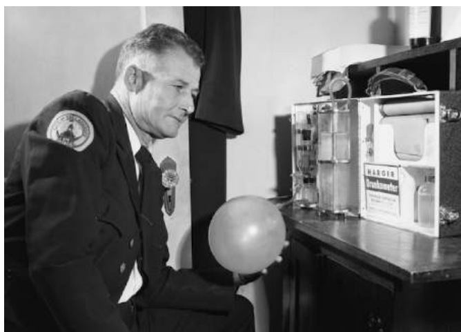
FIGURE 17.16 The Harger Drunkometer was the first breath analyzer, introduced in 1938 to help convict drunk drivers. (credit: “Unidentified police officer with a Harger “Drunkometer” breathalyzer” by Florida Memory, State Library and Archives of Florida/Wikimedia Commons, Public Domain)
