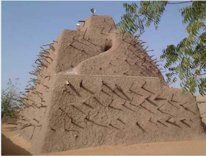
Figure 9.11 | The tomb of Askia the Great built in 1495 in Gao | Note the use of mud (adobe) architecture common in the cities of the Western Sudanic states. People still use the prayer rooms and meeting space at the site.
