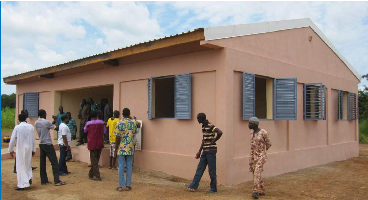
Figure 17.1 The US Army Corp of Engineers opened this community health clinic in the country of Benin in West Africa in 2013. The clinic has waiting, consultation, observation and treatment rooms, and a drug store. (credit: “Pehunco Health Clinic opens” by US Army Corps of Engineers/Wale Adalaku/flickr, Public Domain)
