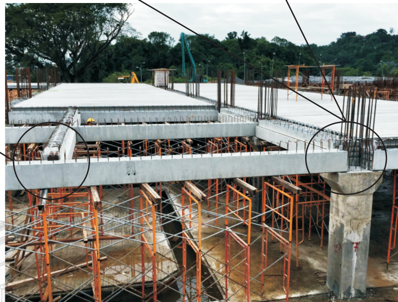
Beam-to-beam connection
