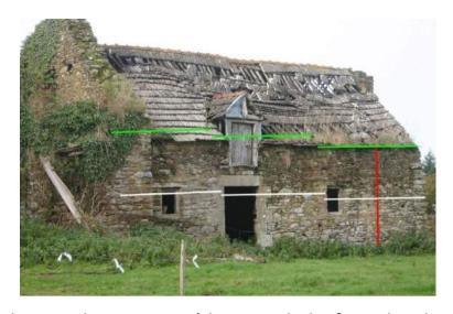
window, we find it is just less than one key measure (shown with the first white line). From the left of that window we measure to the doorway and find that between the left-hand side of the window and the left-hand side of the doorway is one key measure. Now if we go from the left-hand side of the doorway to the left hand window, the left-hand side of the window is about half the key measure. Now try on your own to decide the measurement from from the gutter line to the apex of the roof.
