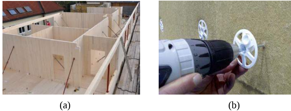
Figure 7 – Building with cut-to-size CLT elements; (a) CLT wall panels erected; (b) Fixing the wood fiber insulation panel to the CLT wall with special screws and a plastic washer.
