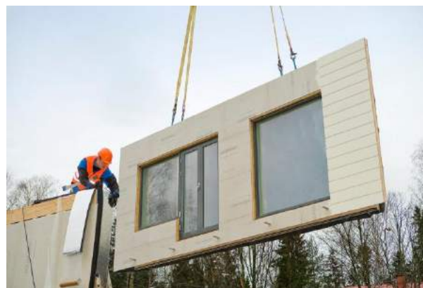
Figure 8 – Assembling of a prefabricated wall element.
