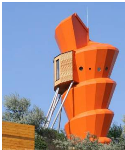
Figure 12 – Spiral Tower pre-fabricated with CLT.
