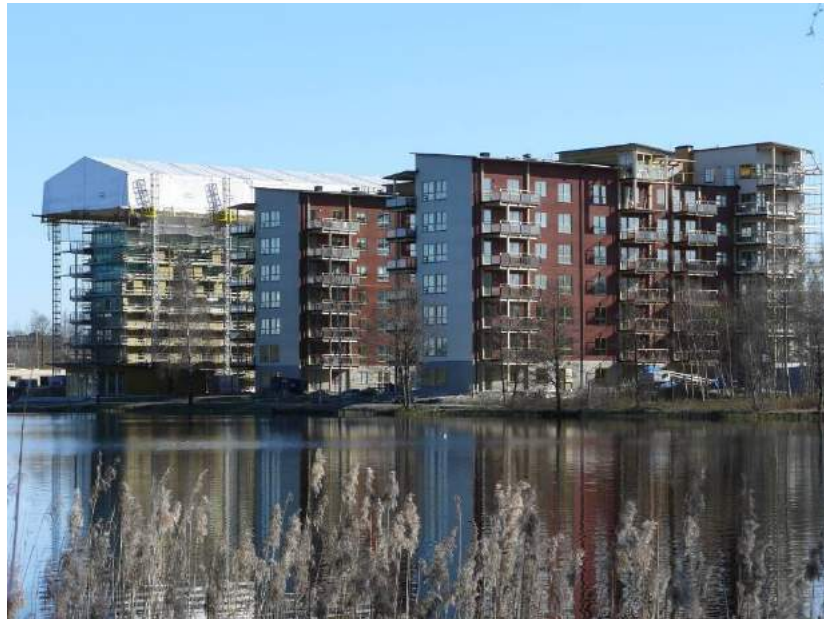
Figure 1 - Limnologen, eight storey residential buildings with timber structure in Växjö, Sweden. To the left, still under construction with a shield for weather protection. (Photo: Växjö University)
