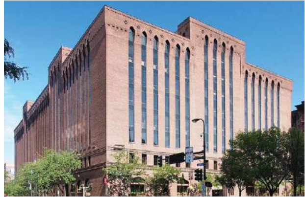
FIGURE 11 Butler building, Minneapolis, United States of America
