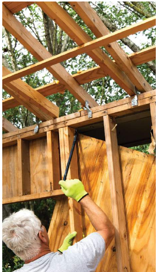
FIGURE 19 Deconstruction for Building Materials Recovery
