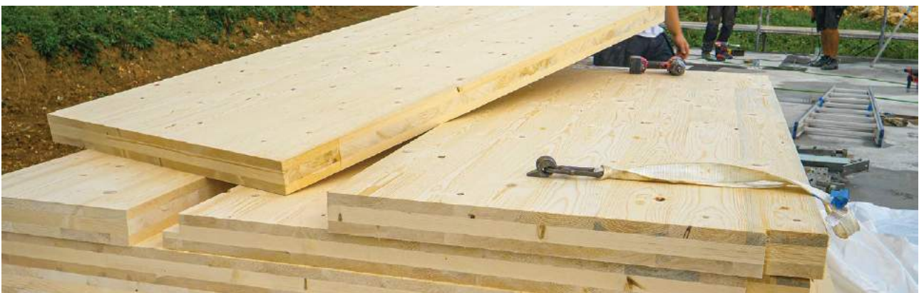
FIGURE 6 Cross-Laminated Timber (CLT)
