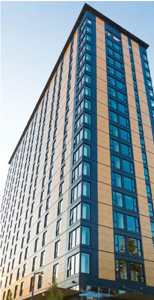
FIGURE 8 Brock Commons, University of British Columbia, Canada
