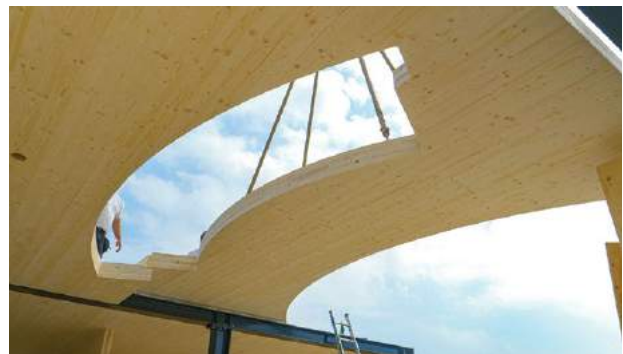
FIGURE 15 Modular Mass Timber Construction
