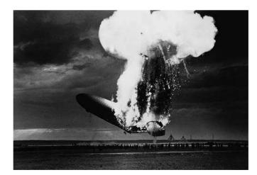
In 1937, a German airship exploded and fell to the ground in a huge fireball as the hydrogen gas which kept it floating ignited and reacted with the oxygen in the air.
