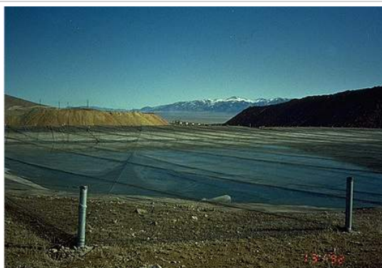
Netted solution pond next to cyanide heap leaching of gold ore near Elko, Nevada (1992).
