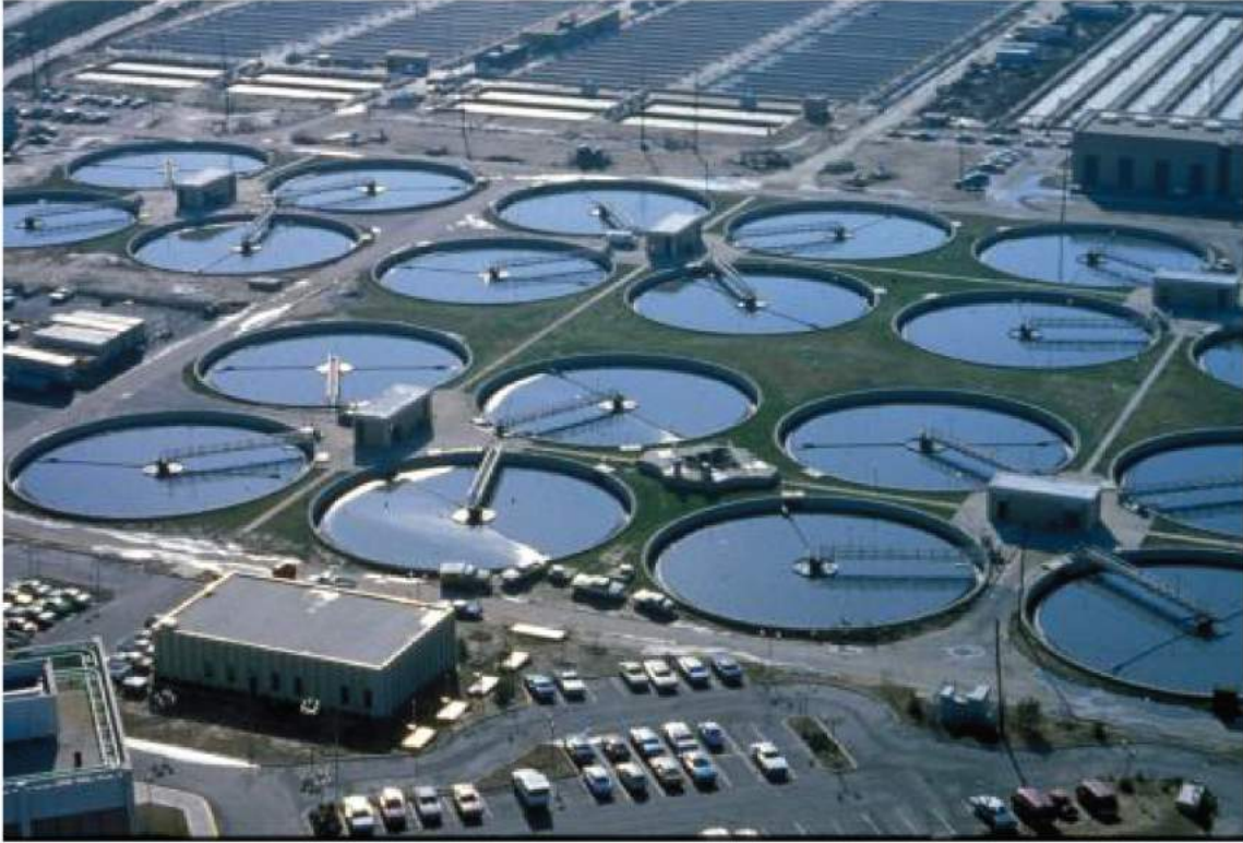
Figure 25.0 Sewage Treatment Plant. (credit: "eutrophication&hypoxia"/flickr.com)
