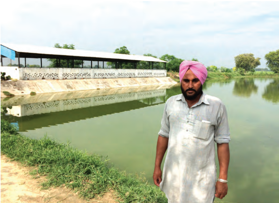
Construction of Pigsty under IFS
