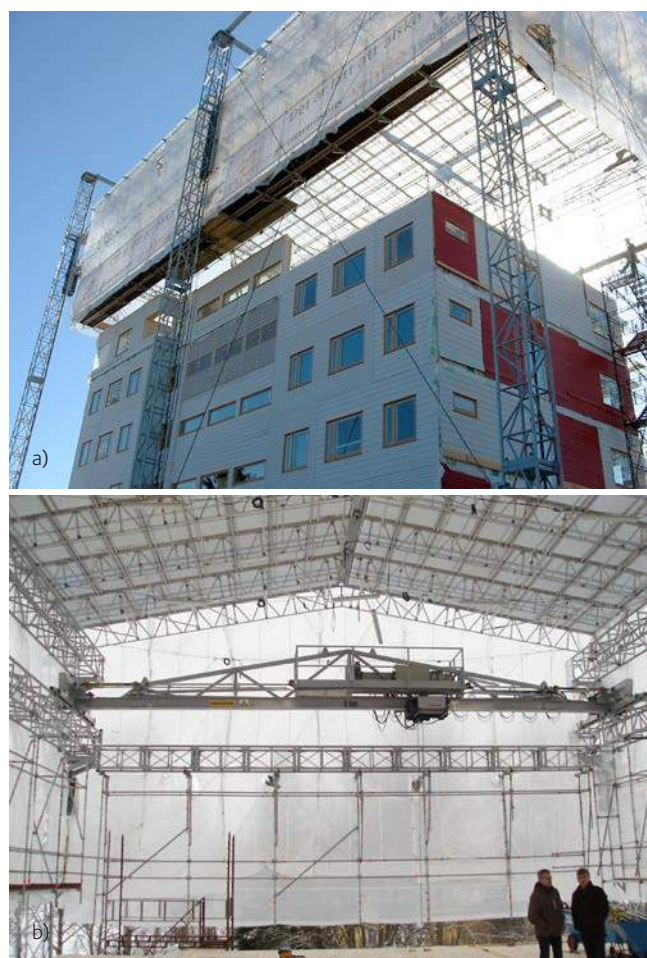
Figure 8.14 a) Movable tent over the whole building. Älvsbacka Strand, Skellefteå. b) Movable tent from the inside with integrated travelling crane.
