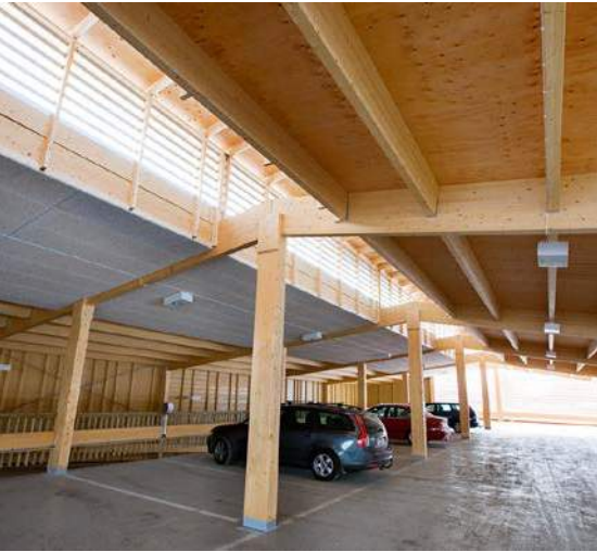
Car park with glulam and CLT frame, Skellefteå.
