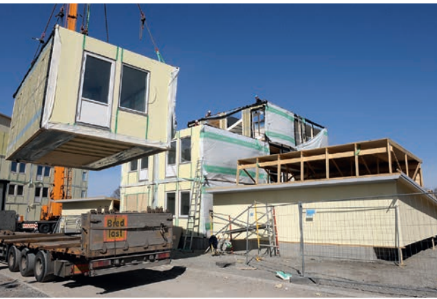
Figure 8.7 Assembly of modular elements
