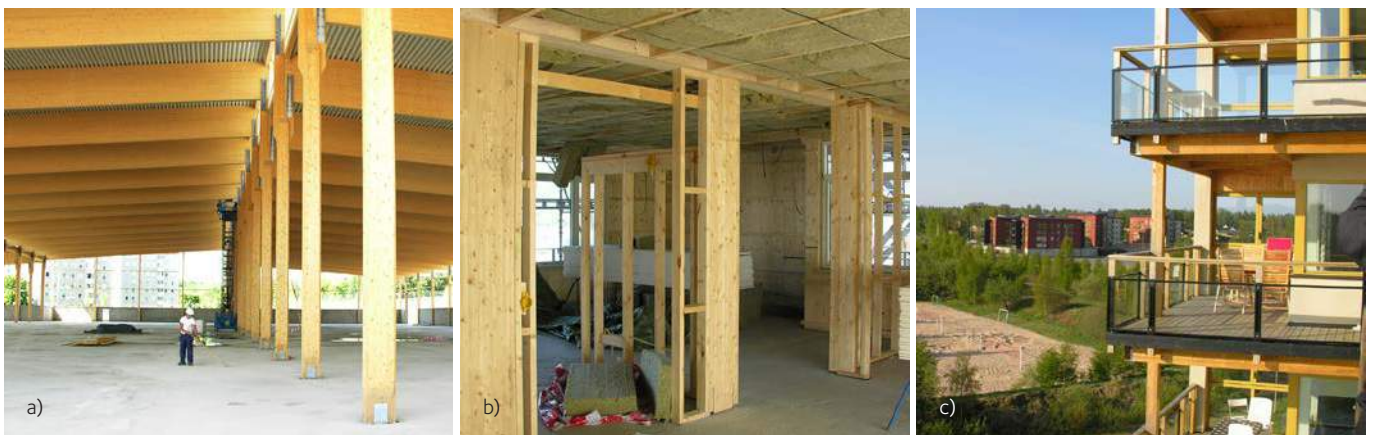
Figure 3.3 Examples of members subjected to compression forces a) Columns in a timber frame, b) studs in a multi-storey timber framed building, c) external columns.
