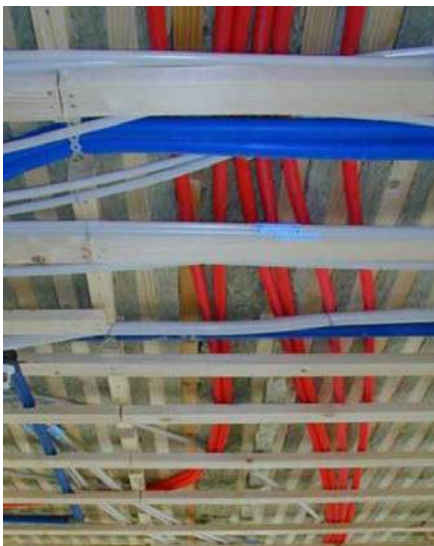
Figure 8.30 a) Ventilation ducts placed in a special shaft. b) Services placed under a floor element before finishing.
