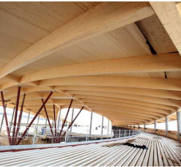
Flat roof made of glulam and CLT.
