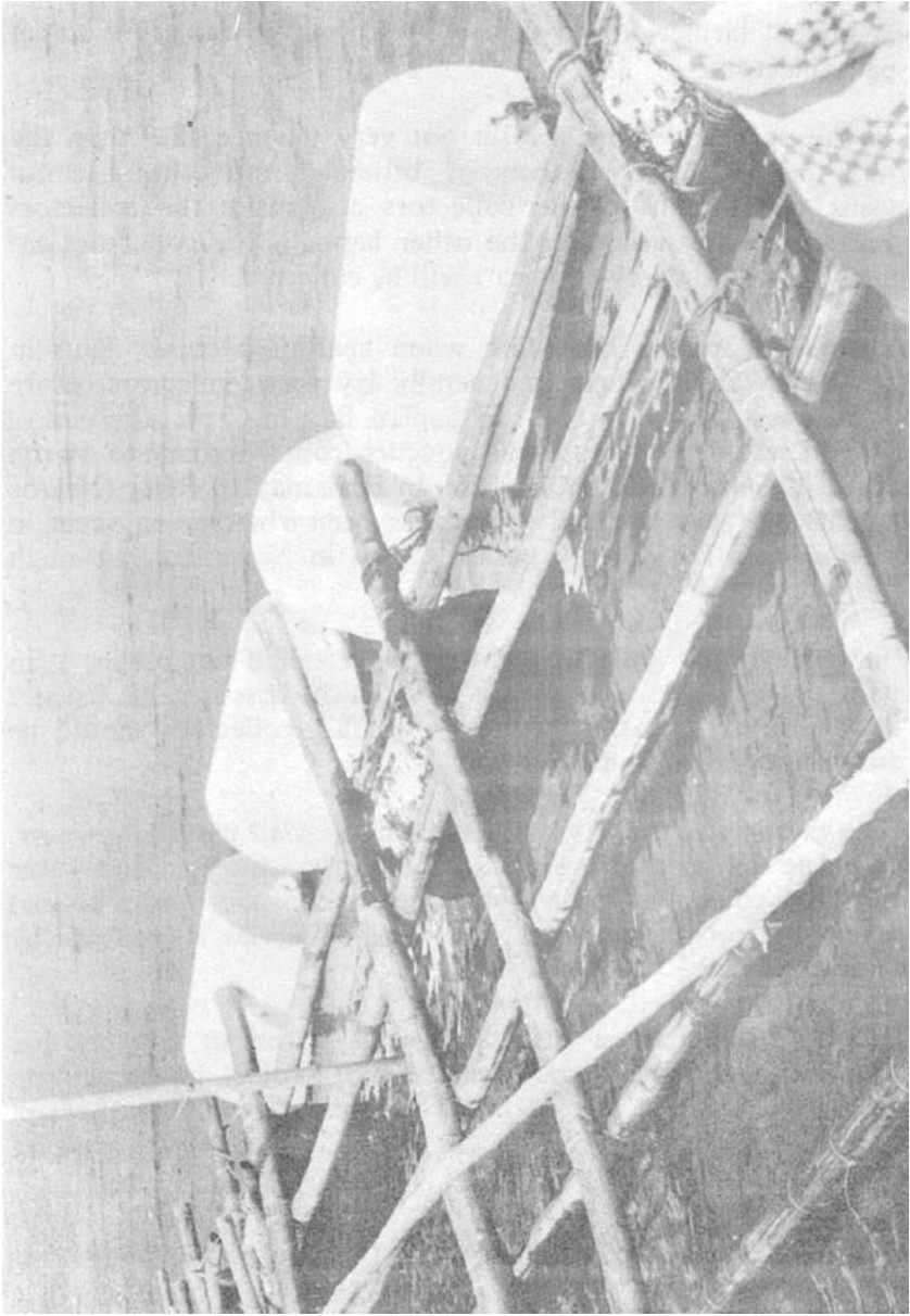
A close up of the floating raft. Note ferrocement buoys used as floats.
