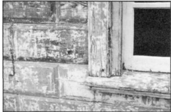
At George Washington's Mount Vernon, a heat plate and a scraper were used to remove the thick layers of paint from the bevelled wooden boards that were cut to imitate dressed ashlar stone. All that is needed before priming is a little light sanding. Photo: Baird M. Smith, AIA, National Park Service files.
