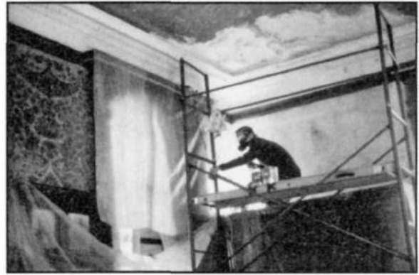
When removing paint, it is always important to take safety precautions. Face masks are specially important when working with lead-based paint that becomes airborne during scraping. Photo: National Park Service files.
