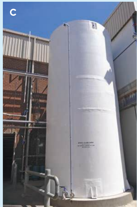
Figure 13: Rivalea Australia's heat recovery system: A. de-superheating heat exchanger, B. heat recovery oil cooler, and C. hot water storage tank
