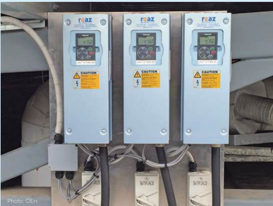
Figure 20: Montague Cold Storage installed VSDs to control evaporator fan speed
