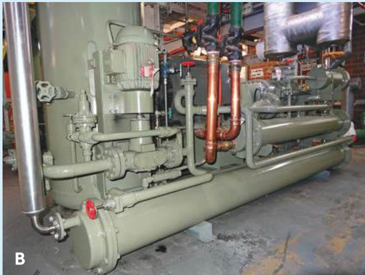
Figure 13: Rivalea Australia's heat recovery system: A. de-superheating heat exchanger, B. heat recovery oil cooler, and C. hot water storage tank
