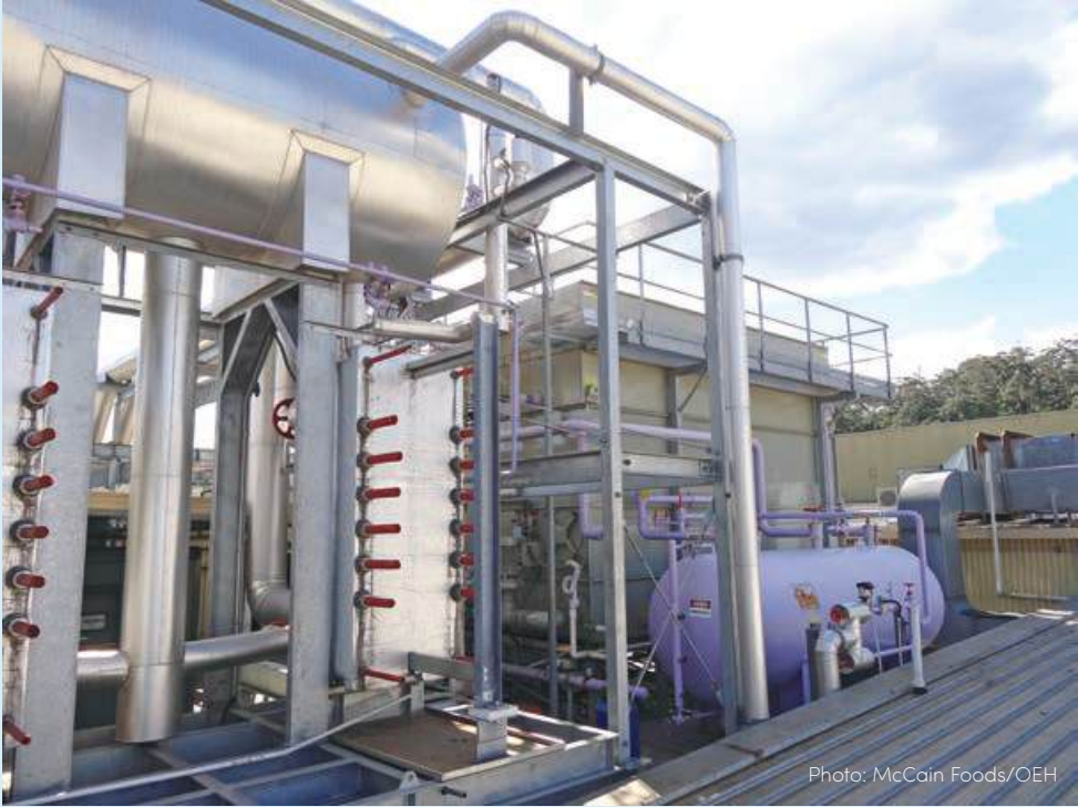
Condensers and plate heat exchangers at McCain Foods in Lisarow
