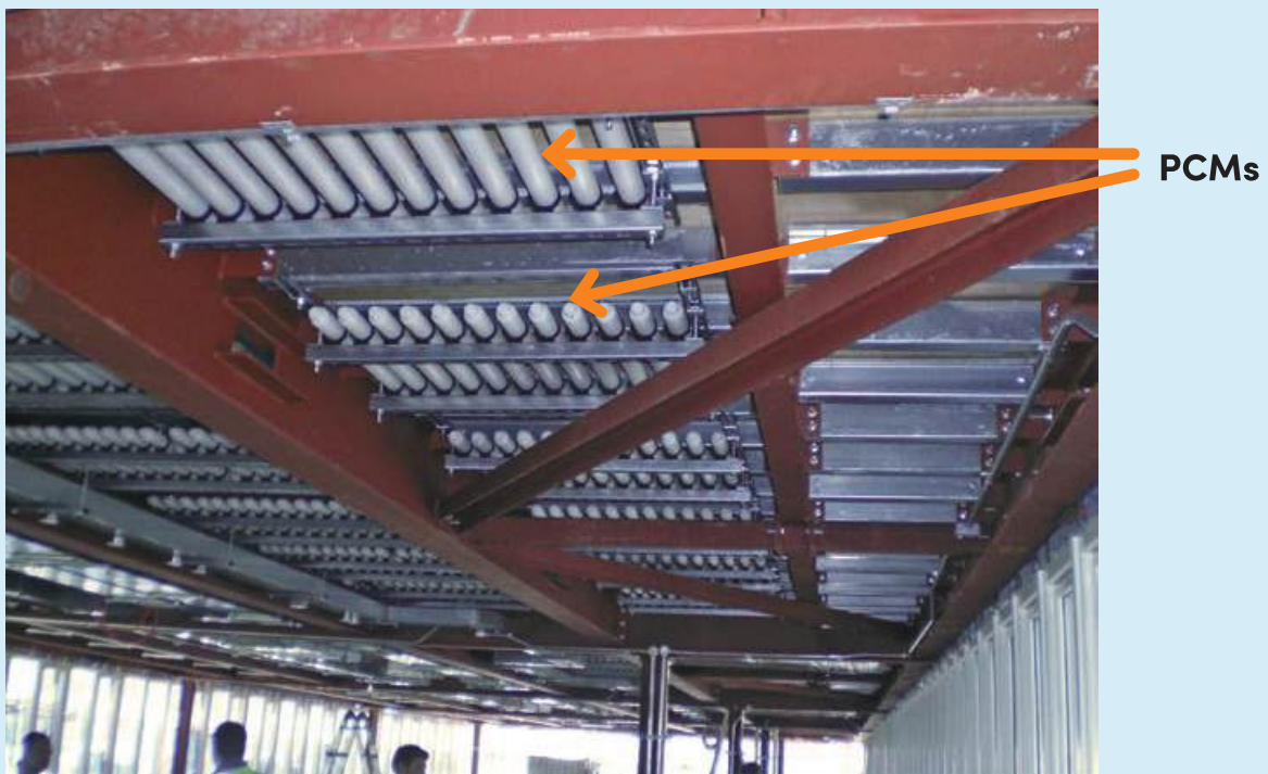
Figure 16: PCMs installed in the ceiling space
