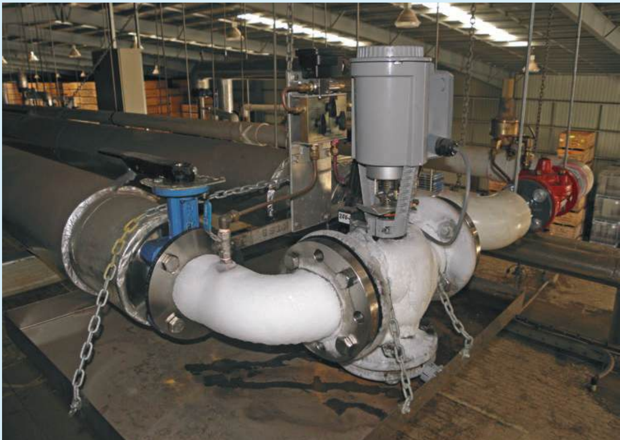
Figure 39: After: a motorised valve installed at the end of the circuit
