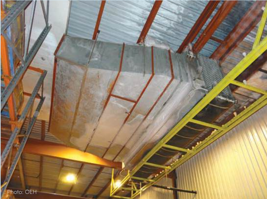
Figure 19: Ammonia evaporators in the Montague Cold Storage cool room
