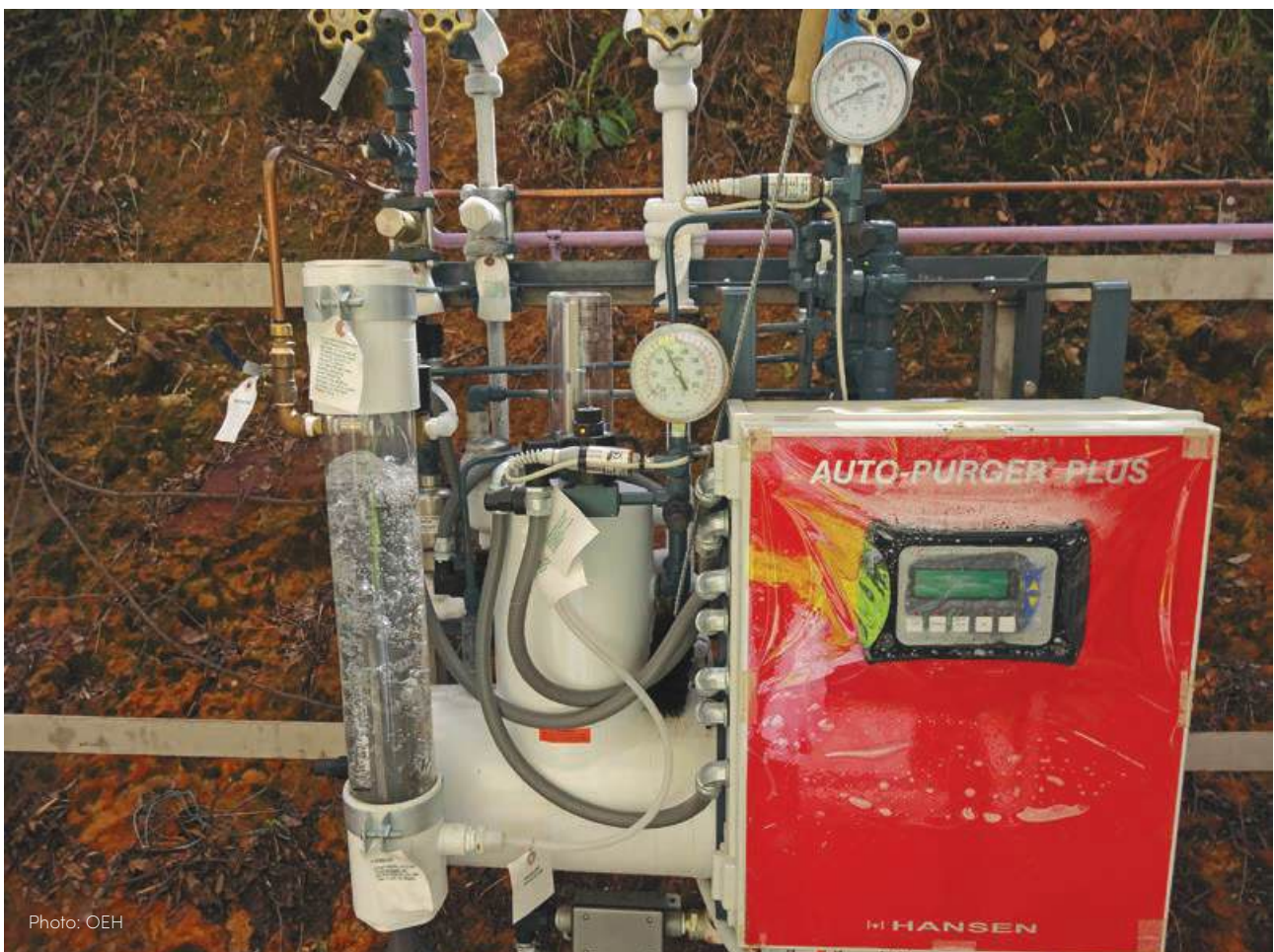
Figure 9: An automatic purger which removes both air and water
