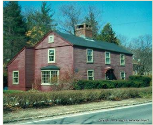
Figure 2-1: New England Large House, Manchester by the Sea, MA. Note the large central chimney and room addition at the rear.
