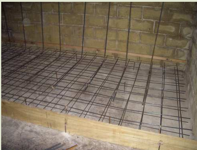
A piece of floor being prepared. 5
