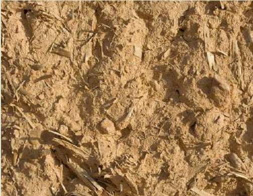
A close up photograph of a mud used to make the wall.
