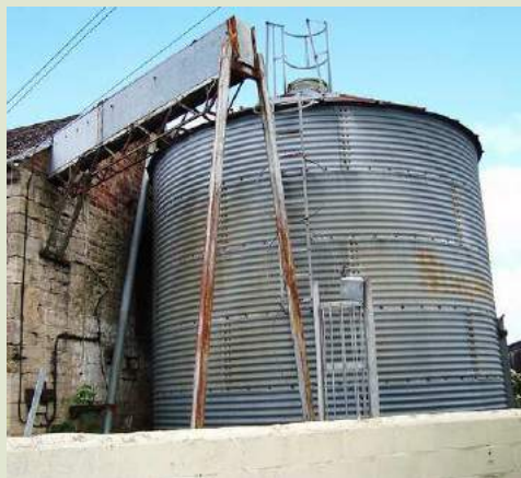
A tank made from corrugated iron. 2
