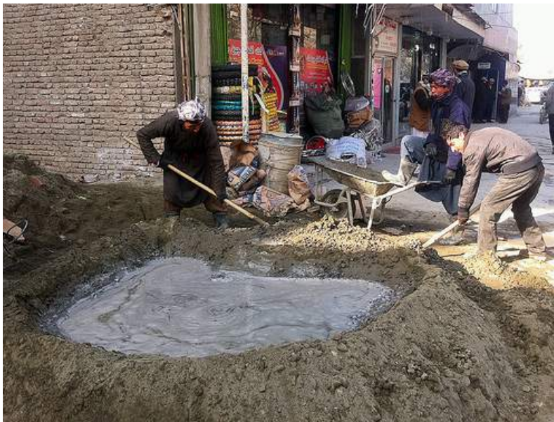
Mixing cement using spades.
