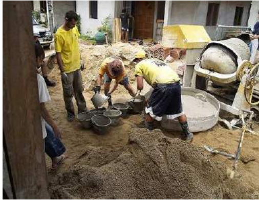
Mixing cement using a mixer.
