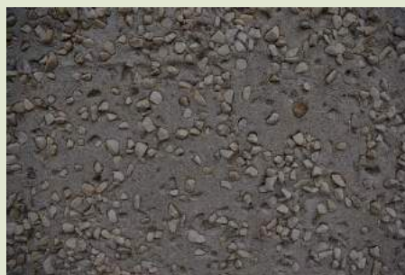
A close up photo of a slab of concrete. 4
