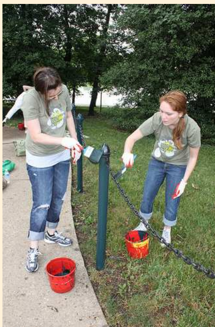
These people are painting the iron poles and fences. 2
