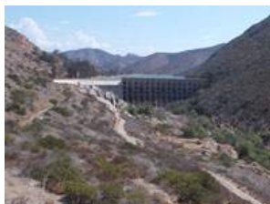
Figure 12.53. Lake Hodges Dam.
