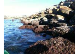
Figure 12.52. Rip-rap was used in the construction of the breakwater (Oceanside Harbor).
