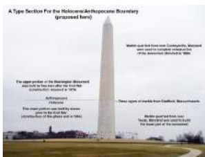
Figure 2.81. The Washington Monument is a possibly a good choice for a type section for the Holocene/Anthropocene Boundary . The lower part of the monument was built (by slaves) before the Industrial Revolution began. The upper part of monument was completed in a second construction phase after the Civil War (by free men) after the Industrial Revolution was well in progress.
