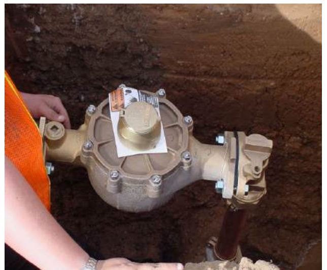
Installation of a new customer water service line.
