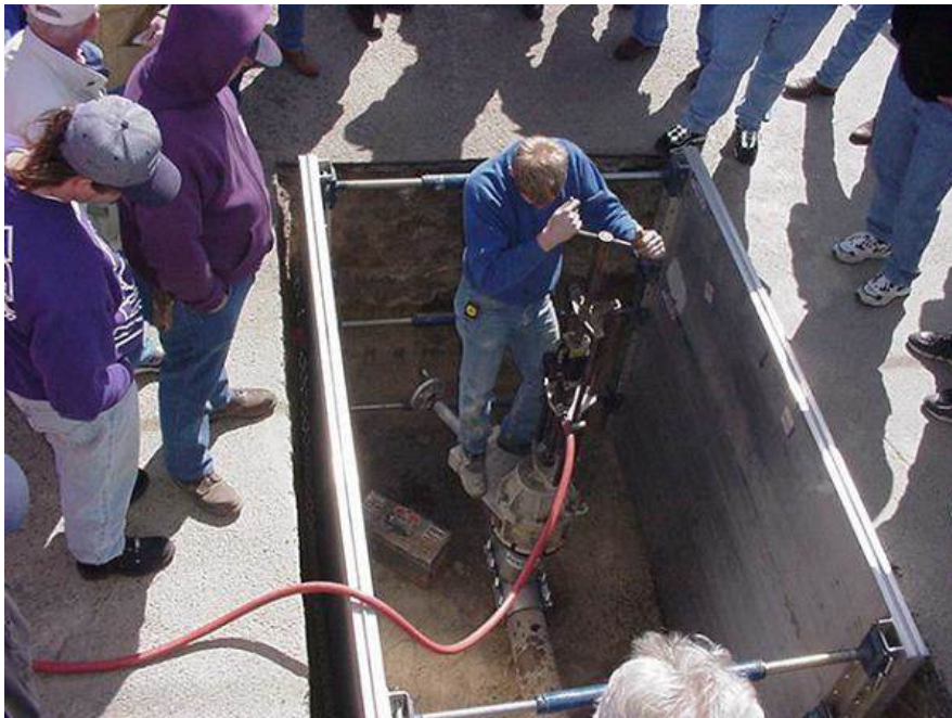
Hydro-Stop valve insertion machine
