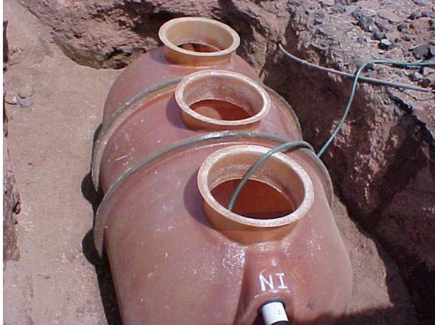
Three Compartment Grease Interceptor
